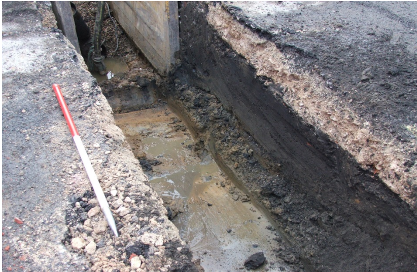
Figure 3: Drainage trench, looking west
