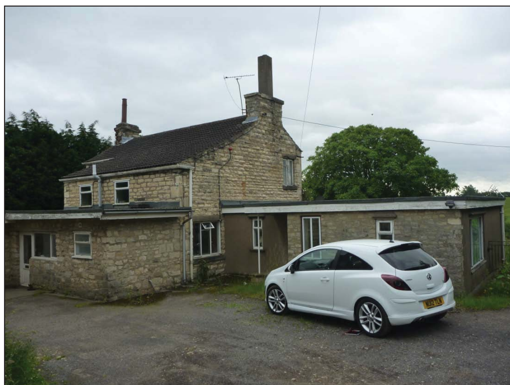
Plate 3 The north and west elevations of the house and its modern extensions, looking south-east
