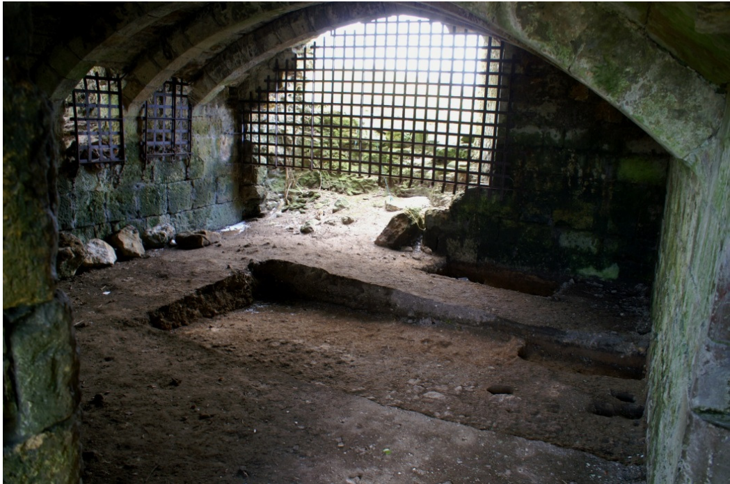
Figure 4: General view of Trench 1 from the entrance to the chamber
