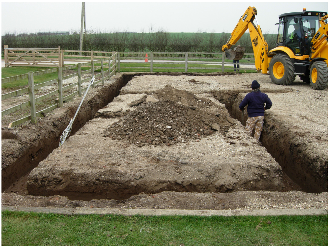
Plate 2 The foundation trenches for the new building viewed from the east
