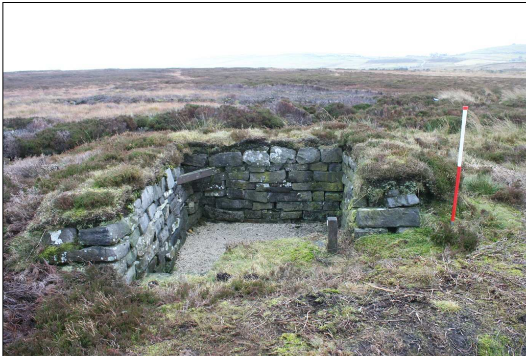
Plate 14: Example of a drystone-constructed shooting stand (Site 47)
