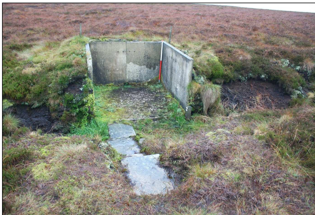
Plate 15: Example of a concrete slab-constructed shooting stand (Site 8)
