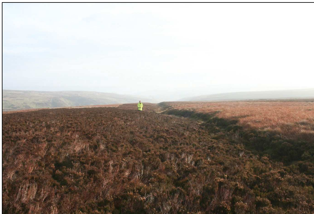
Plate 10: Leat system (Site 77) draining Cranberry Moss into a dam at Stoney Grooves mine (Site 67), looking east-south-east
