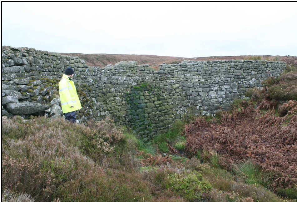
Plate 9: Drystone revetment above the outfall on the dam wall (Site 67), looking north-west
