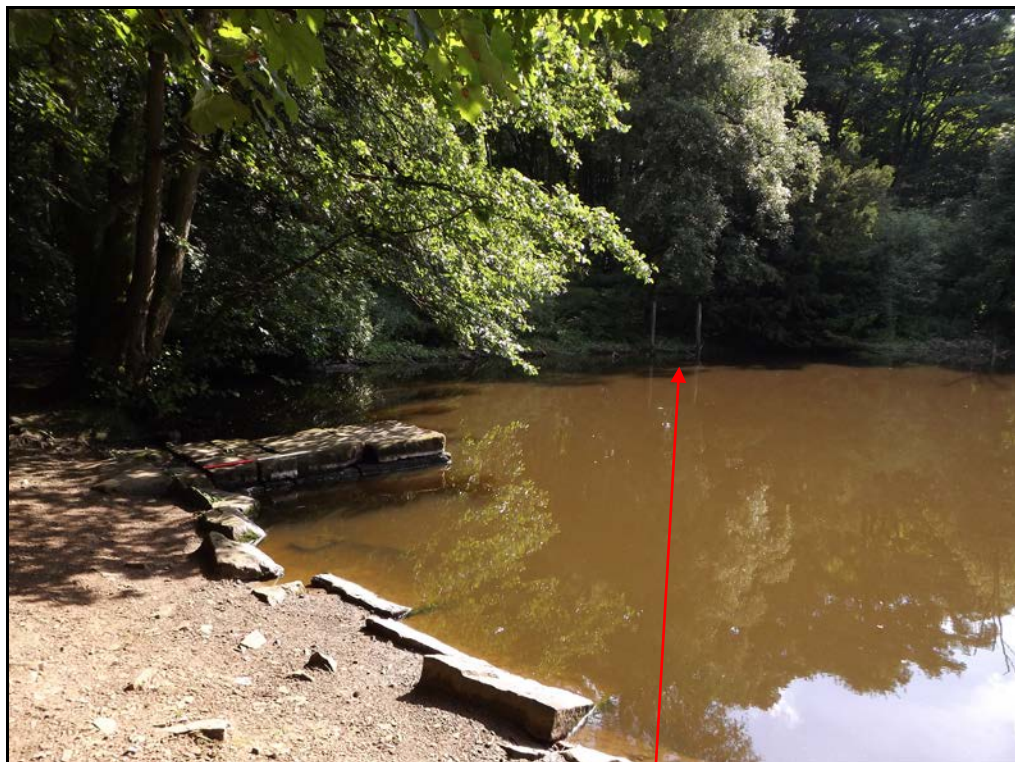
Figure 13. Edge of dam, jetty and remains of boat house
