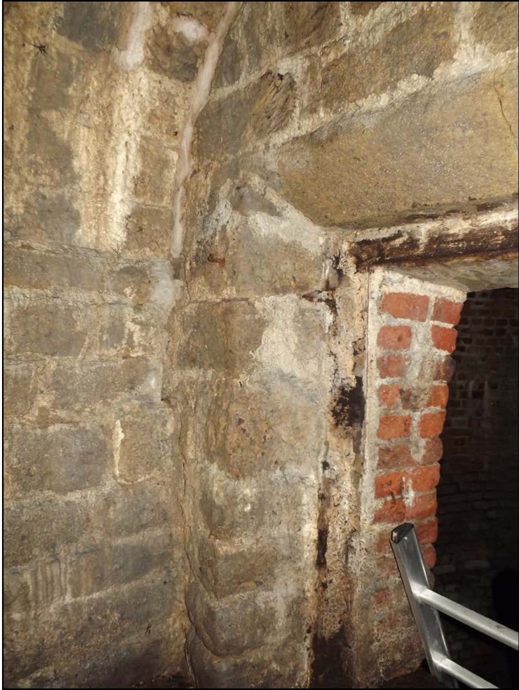
Figure 7. Detail of butt joint between stone and brick work, looking NW
