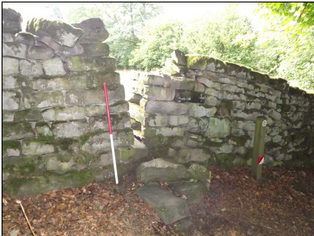
Figure 28. Stone stile along western boundary, showing narrowing of opening, scale 1m, looking NW
