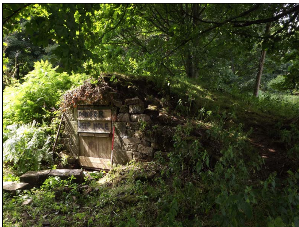
Figure 6. Stone built entrance to ice house, looking NW, scale 1m
