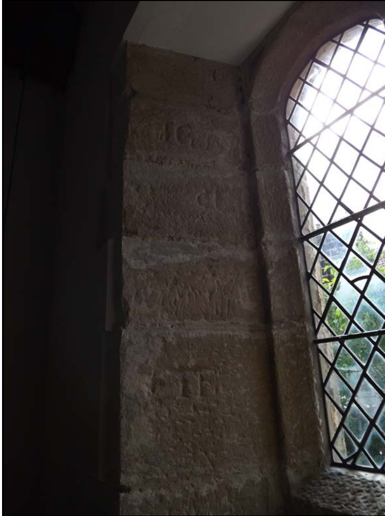
Figure 33. Graffiti in the window reveal on the south side of the chapel
