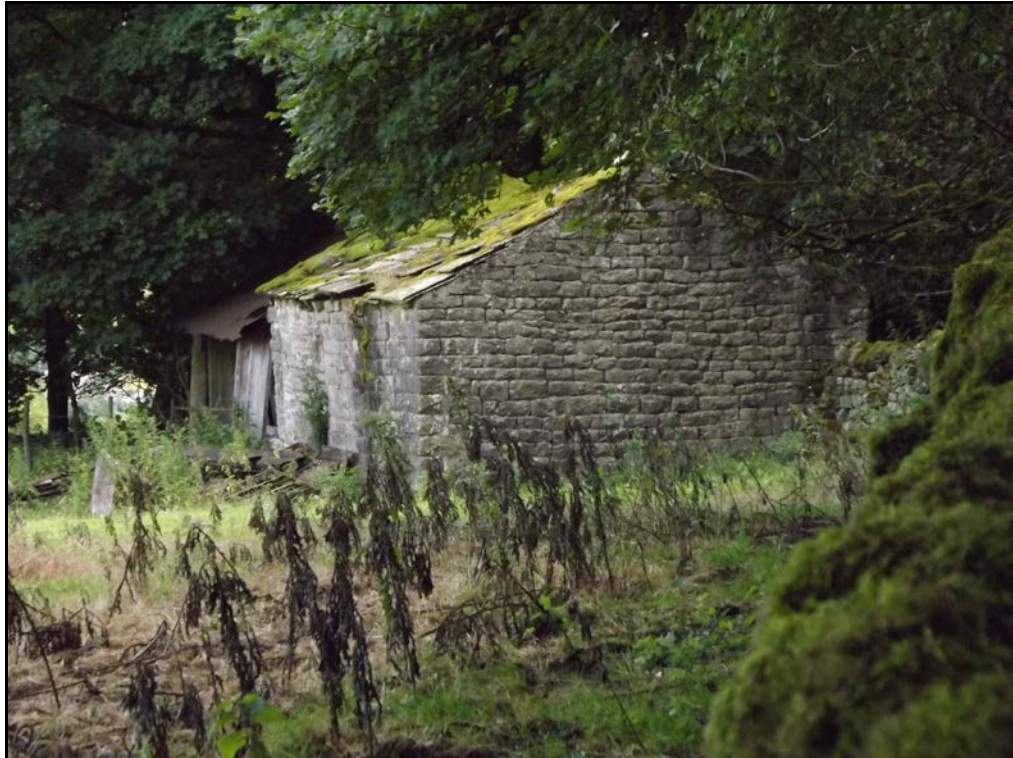
Figure 30. Stone built barn on the northern boundary, looking east
