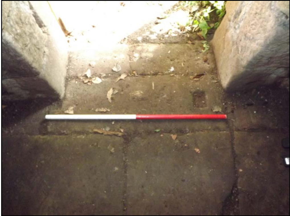
Figure 8. Remains of earlier door frame in flags, scale 1m
