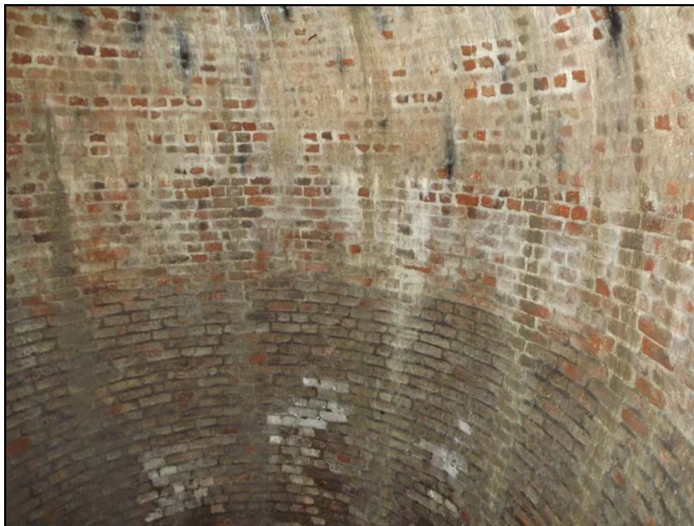
Figure 5. Part of brick lining of ice house
