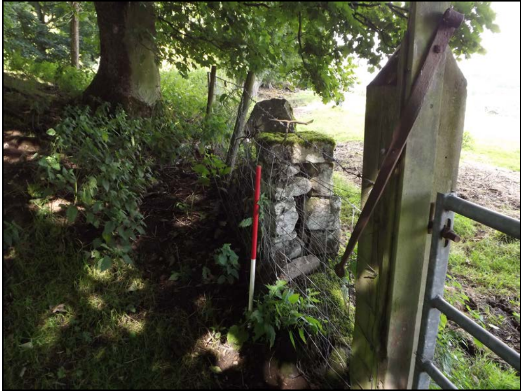
Figure 9. Possible wall end adjacent to ice house, note re-used iron strap hinge of possible 17/18 th century date.
