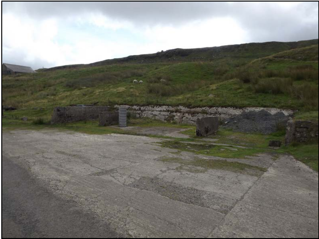
Figure 14. Coal Bunkers – Site 2, looking south-east
