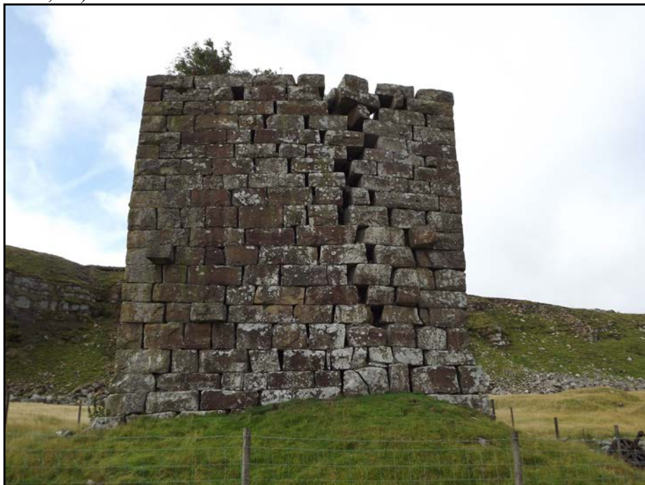
Figure 25. Stone tower for winding gear, looking north-east
