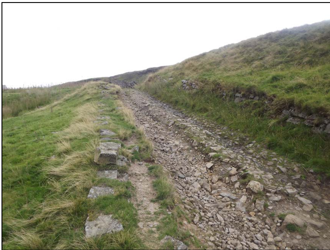
Figure 4. Old Middlesmoor Road with remains of cobble surface and possible trod on left hand side
