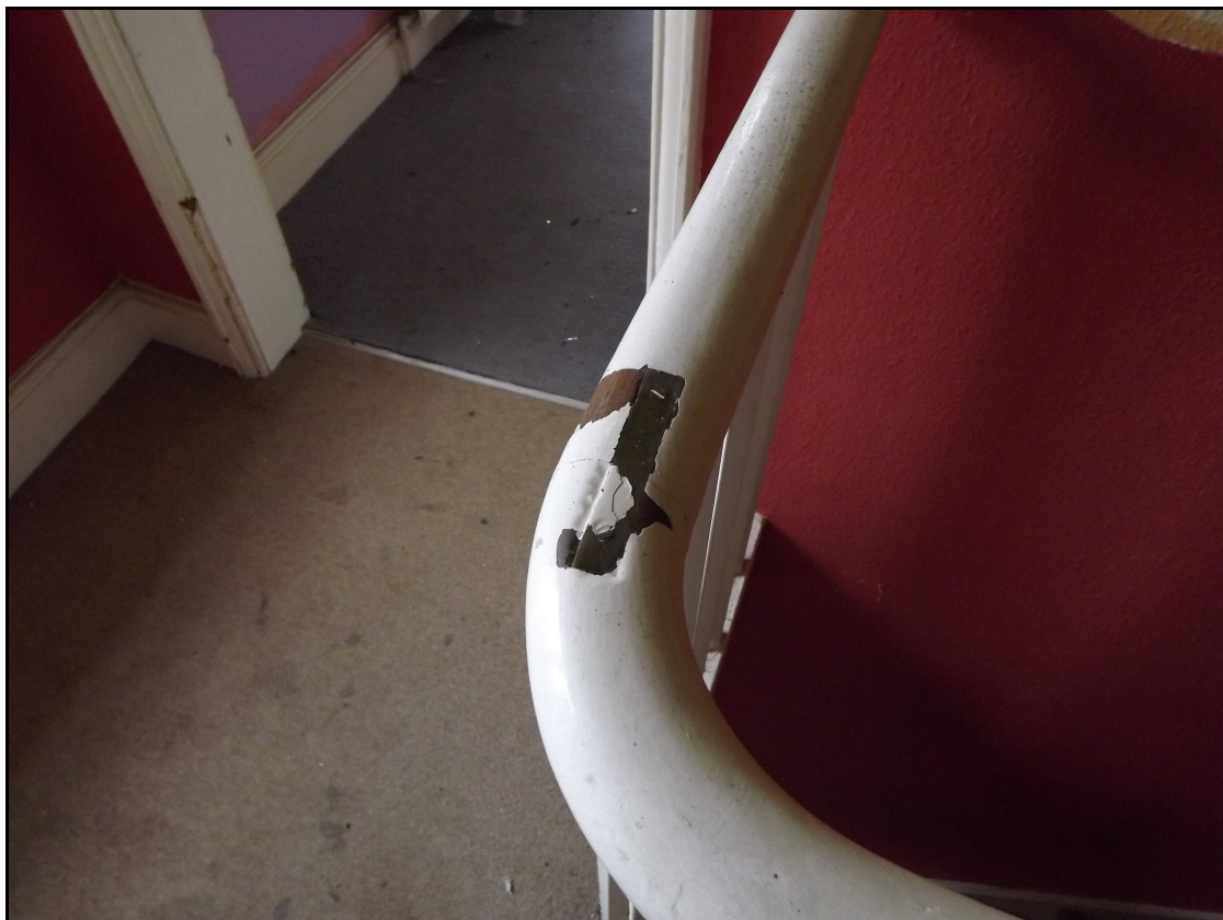
Plate 15. Detail showing copper alloy connection plates for handrail of banisters
