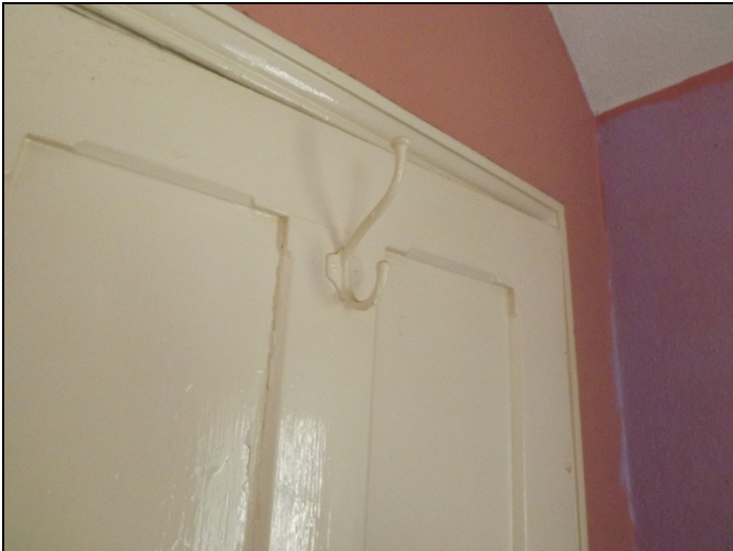
Plate 10. Original coat hook on back of main bedroom door
