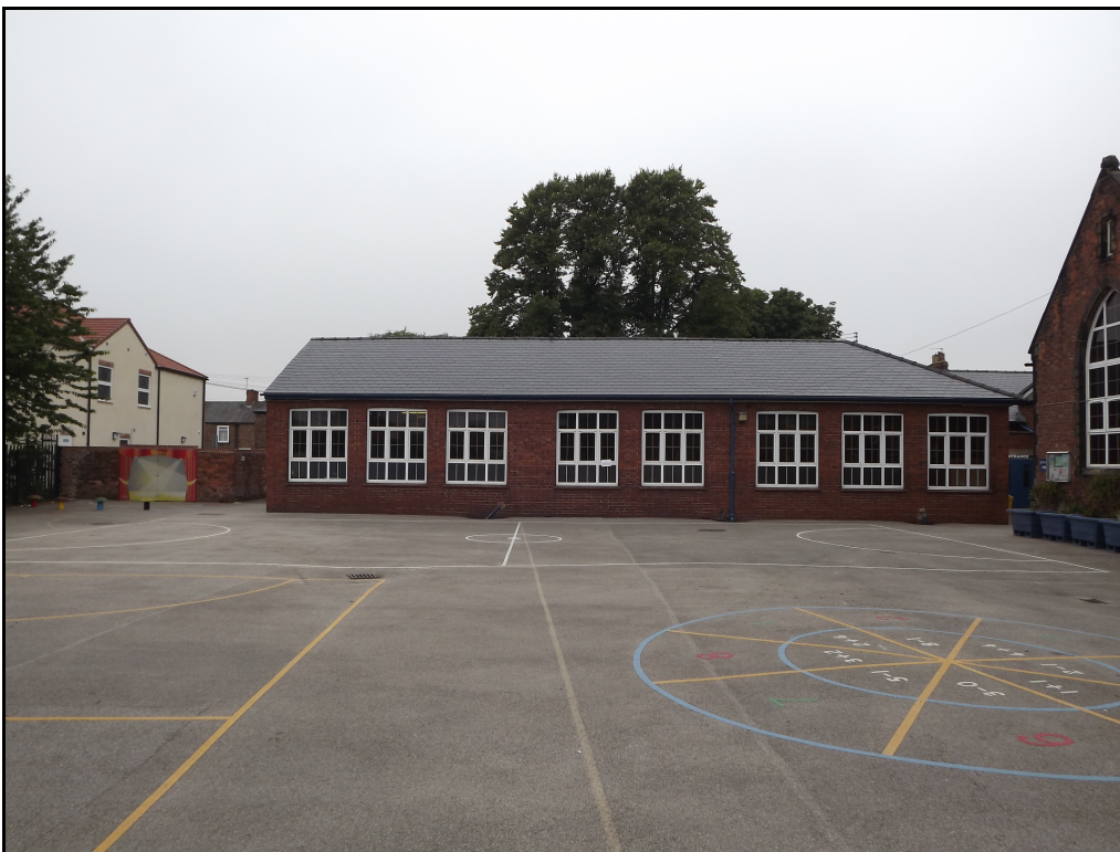
Plate 24. Eastern elevation of the Seniors Classrooms, looking west
