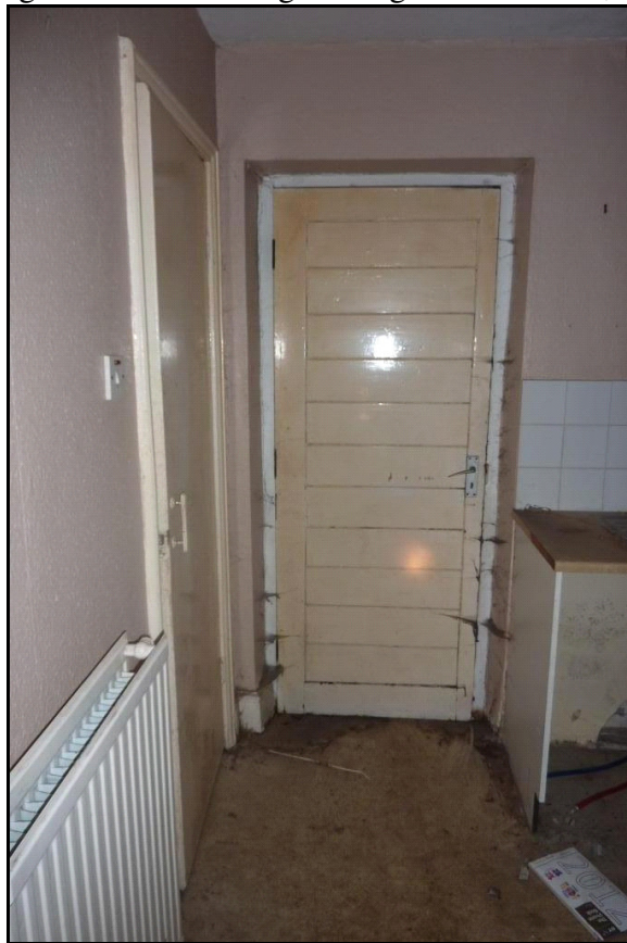
Plate 13. Inside of back door to house, looking ESE
