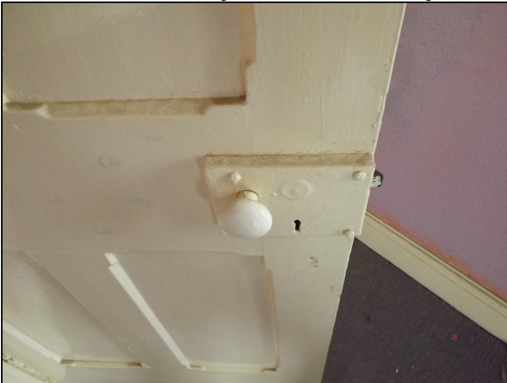
Plate 9. Original lock on main bedroom door, note decorative chamfer on door panels
