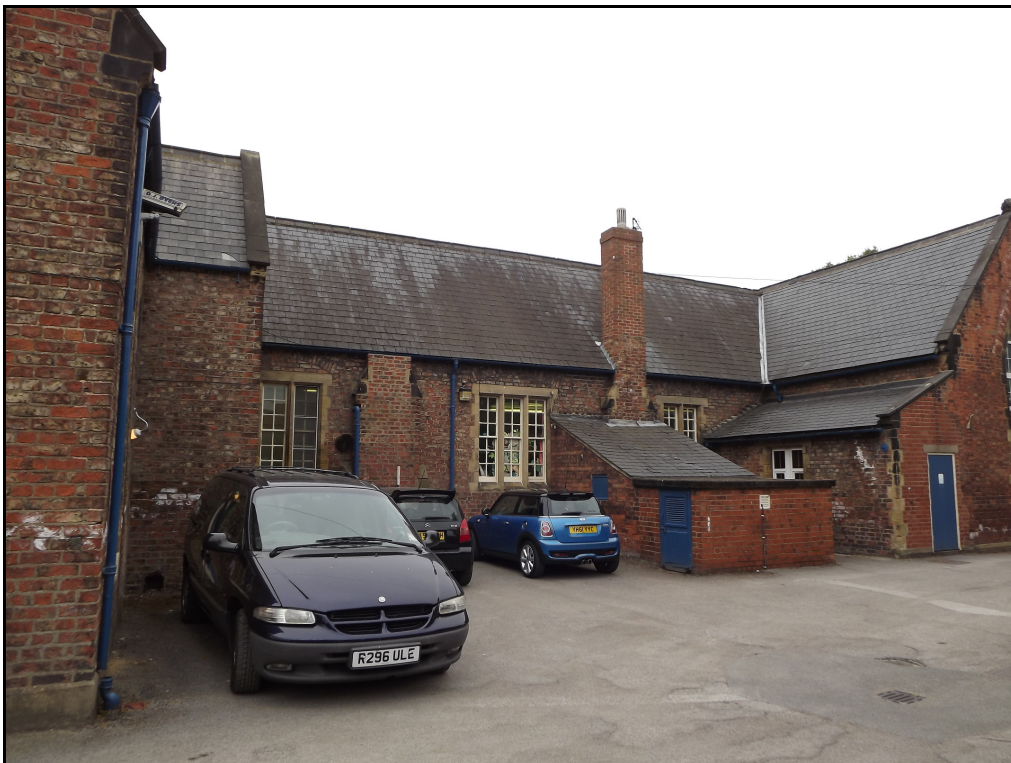
Plate 16. Northern elevation of main school building, looking south-west
