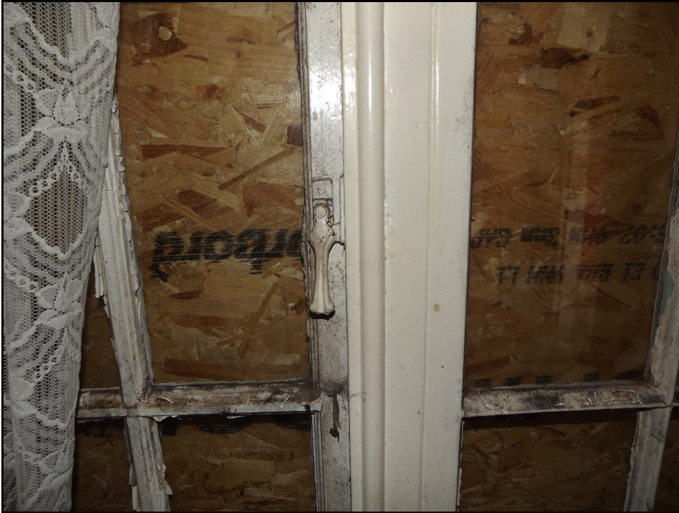
Plate 12. Detail of ?original window fitting. Dining room window, looking WNW
