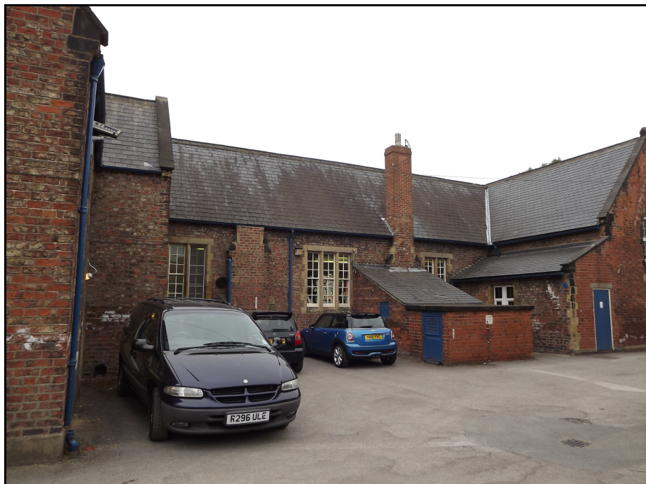
Plate 22. Northern addition to main building, looking south-west
