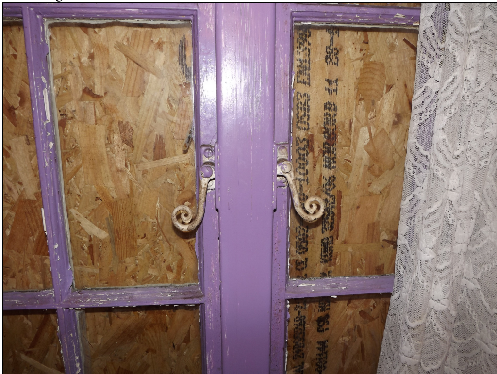
Plate 11. Detail of later window fittings. Lounge window, looking WNW
