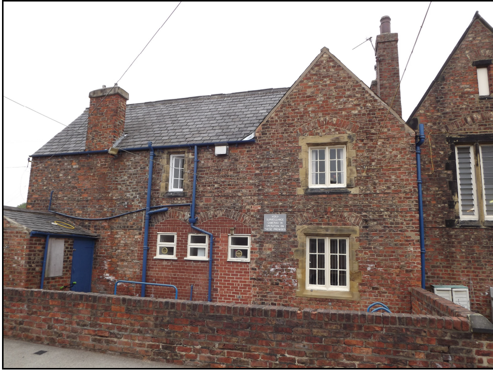
Plate 5. Blocked openings on the eastern elevation of the School Masters House
