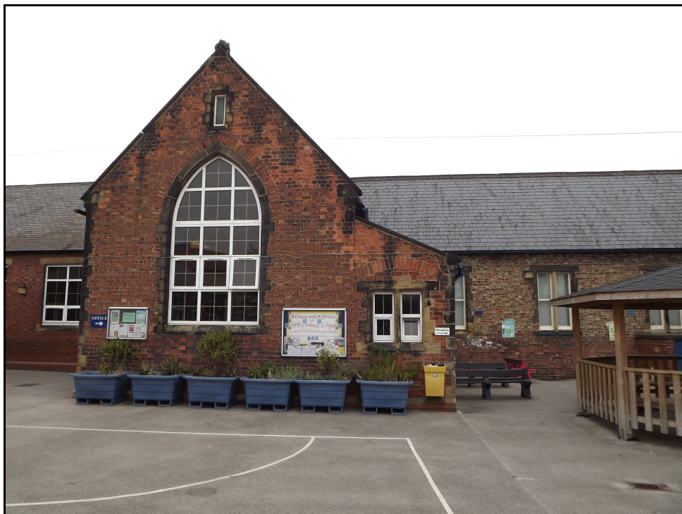
Plate 18. Southern elevation of main school building, looking north
