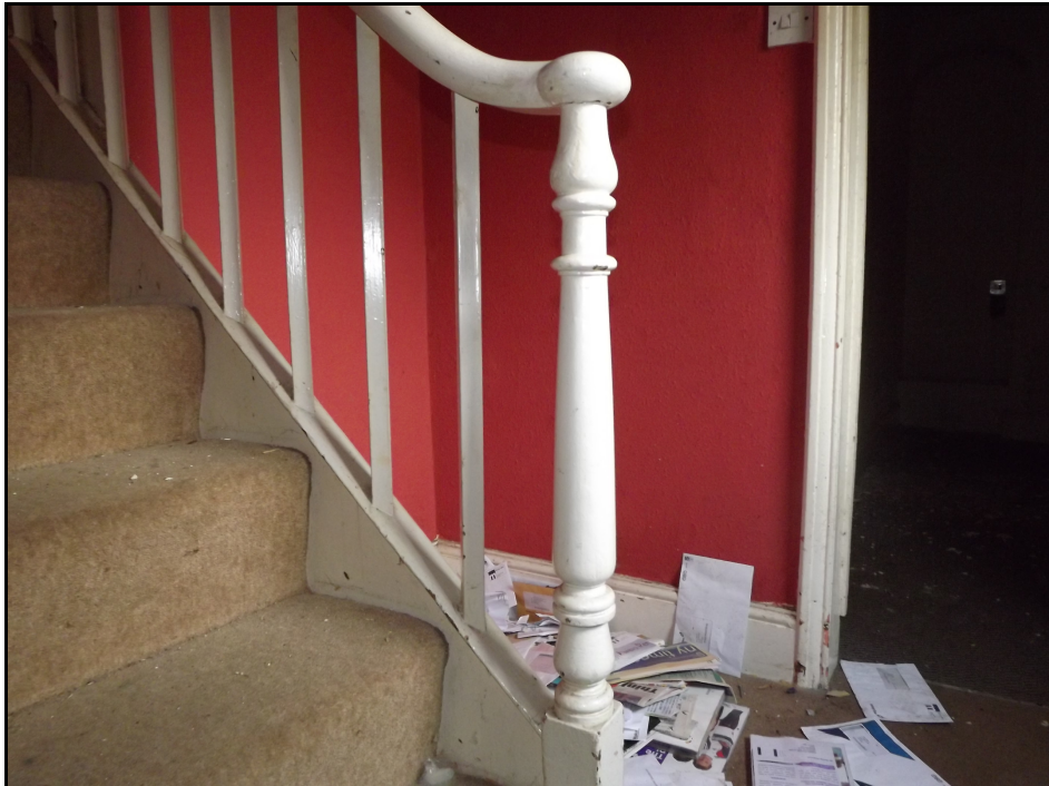
Plate 14. Detail of the bottom of the stairs showing newel post and spindles
