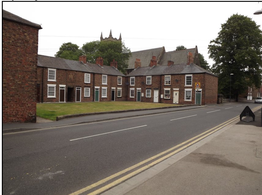
Plate 32. Nos 46-72 New Lane, Grade II Mid 19 th century housing to the south-west of the school (Asset 13)
