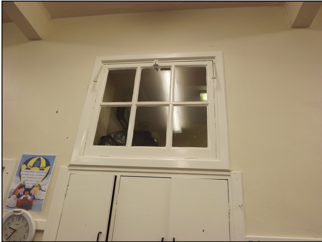
Plate 29. Internal glazing at eastern end of building
