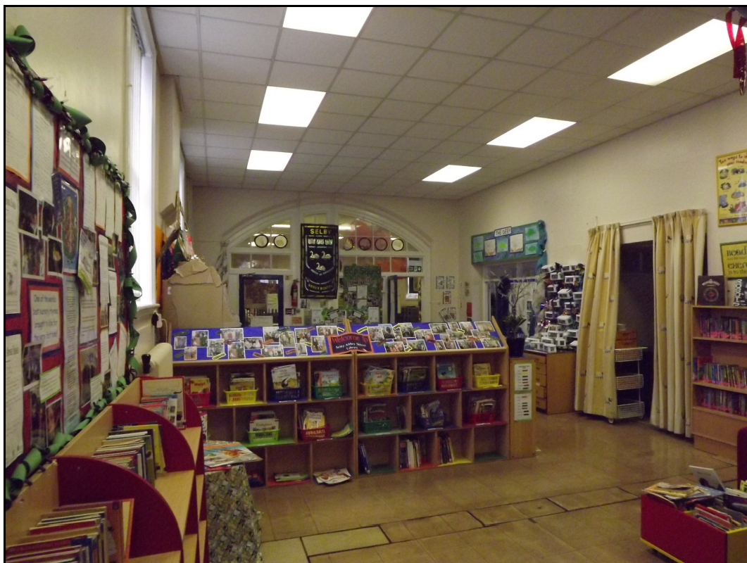
Plate 19. South range of the main school buildings, showing the glazed partition between the south and west Ranges
