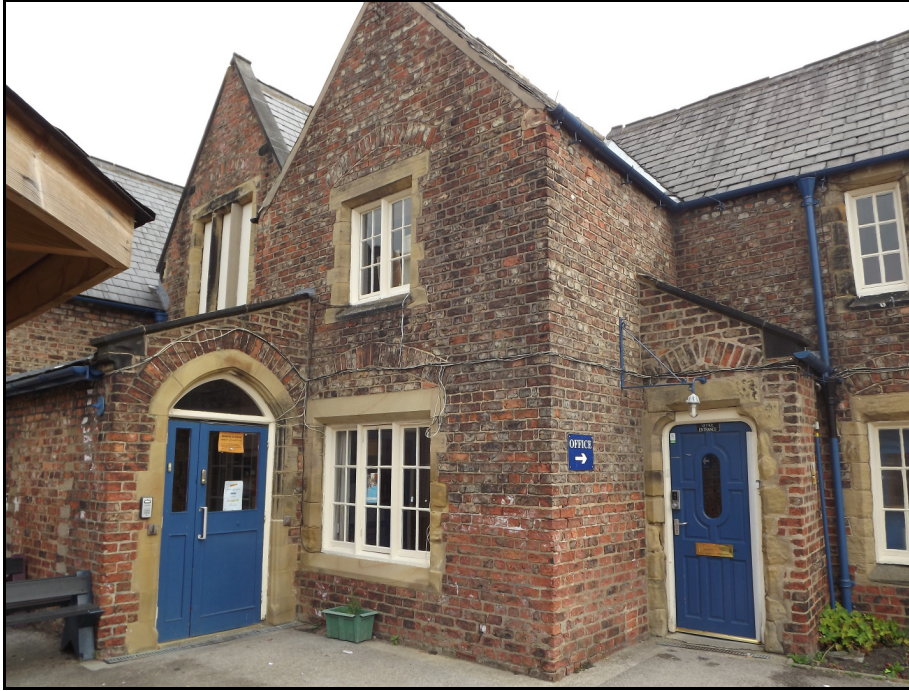
Plate 1. Part of the School Masters House of the 1858 National School showing original construction materials, looking north-east
