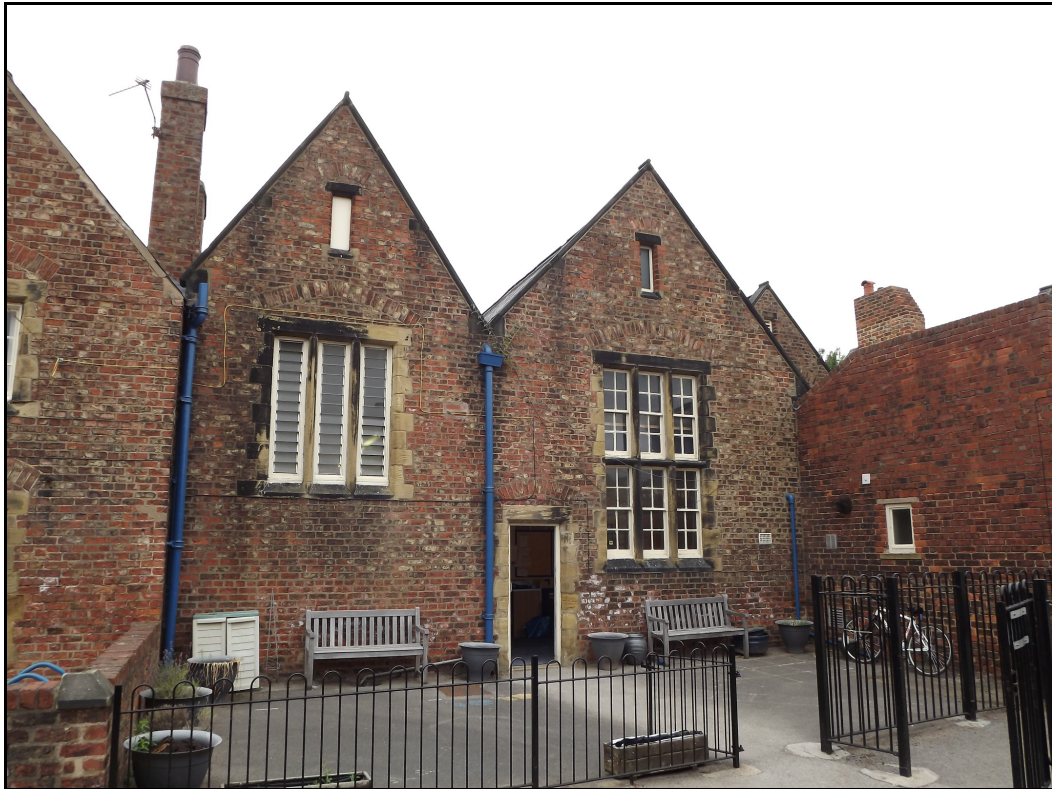
Plate 17. Eastern elevation of main school building, looking north-west
