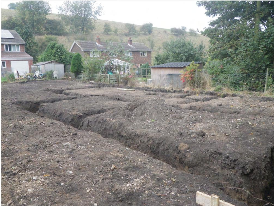
Plate 5. Plot 3. Facing North-west.
