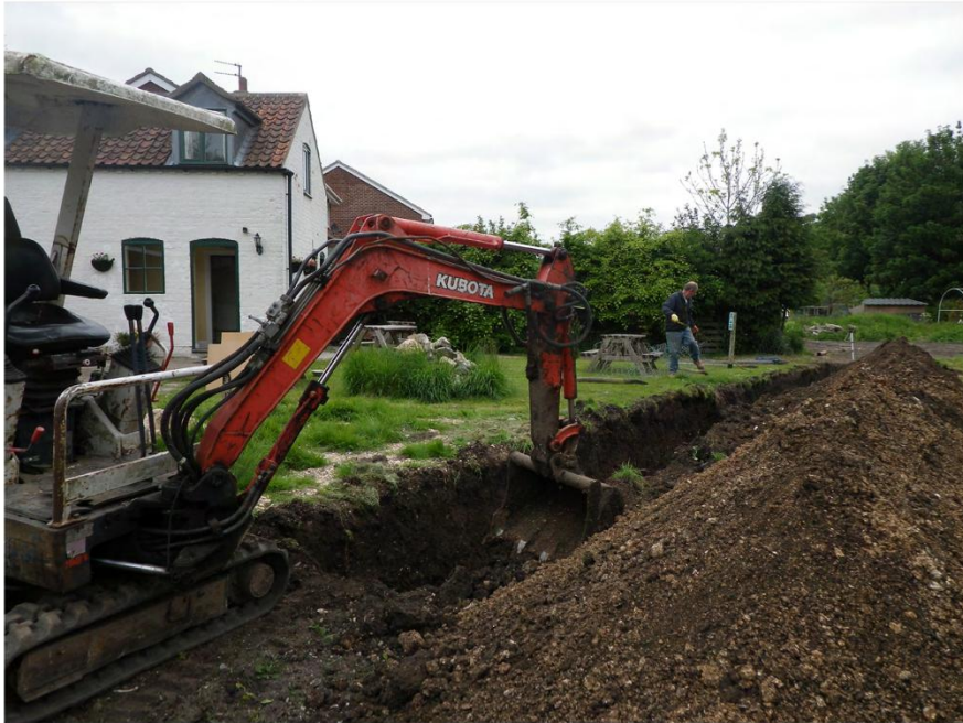
Plate 1. Drainage Trench. Facing North-east.
