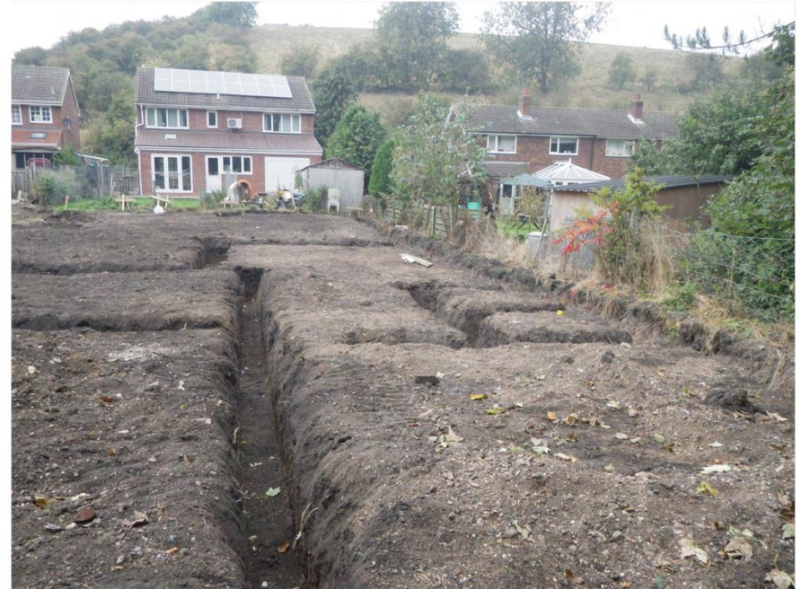
Plate 4. Plot 3. Facing North-west.
