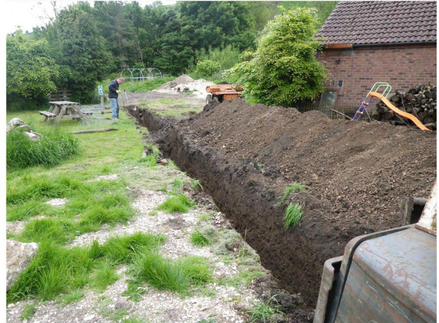
Plate 2. Drainage Trench. Facing South-west.
