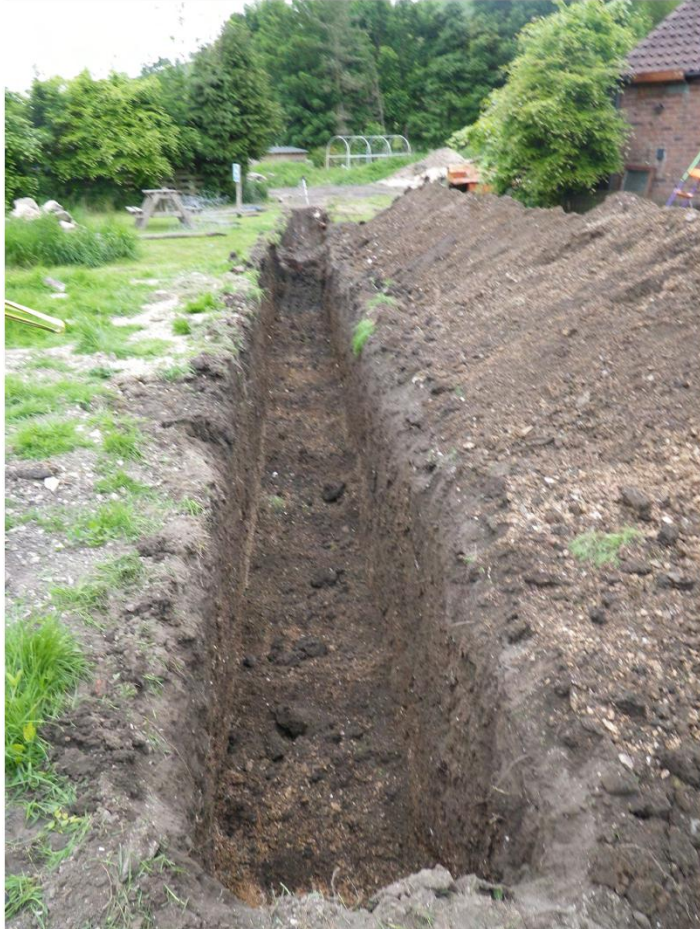
Plate 3. Drainage Trench. Facing South-west.
