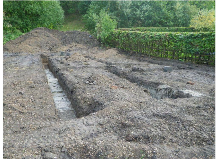
Plate 6. Plot 1. Facing South-east.
