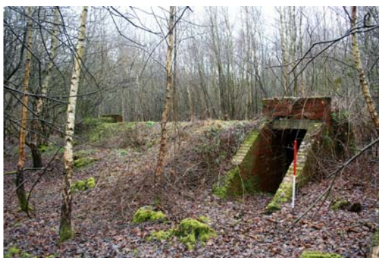
Plate 27: Air Raid Shelter, Site 49
