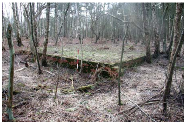
Plate 41: Brick Platform, Site 148
