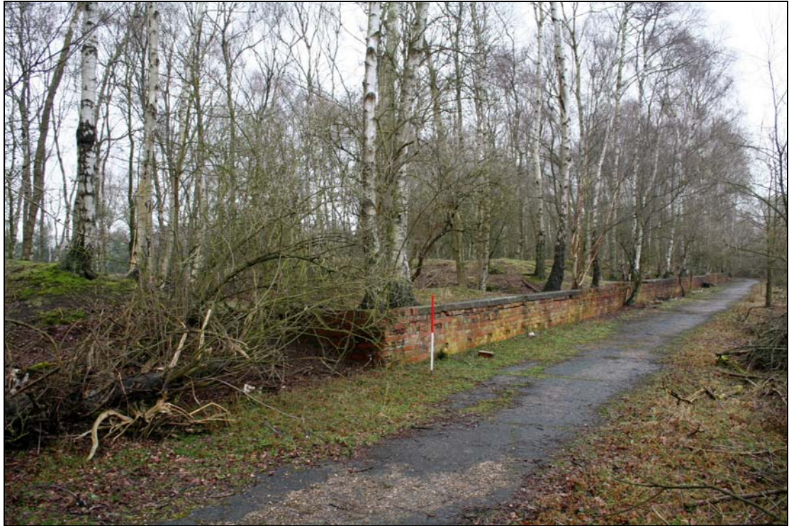
Plate 14: High explosives bomb store – Phase II, Site 88
