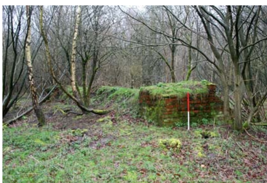
Plate 23: Air Raid Shelter, Site 30
