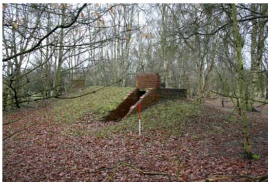
Plate 38: Air Raid Shelter, Site 105
