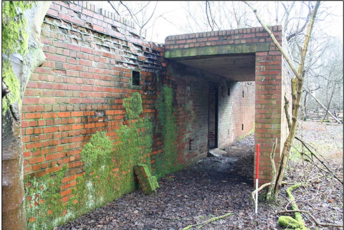
Plate 16: Central entrance and blast wall on small arms ammunition store, Site 270
