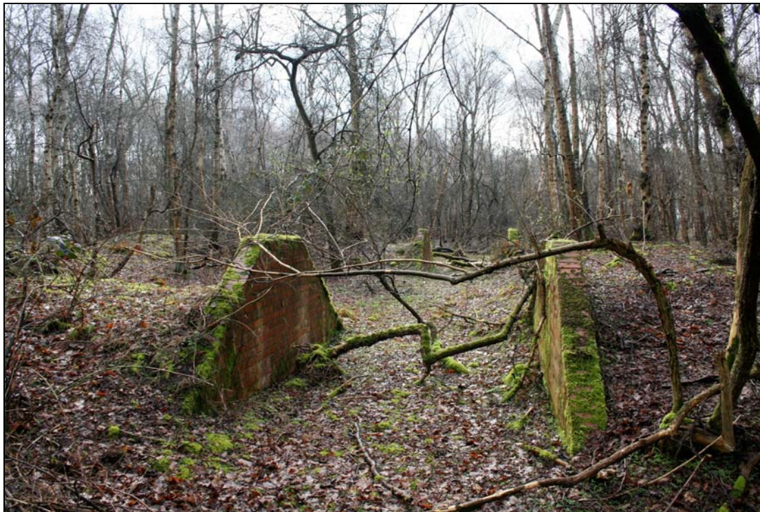
Plate 13: Blast banks for a high explosives bomb store – Phase I, Site 272
