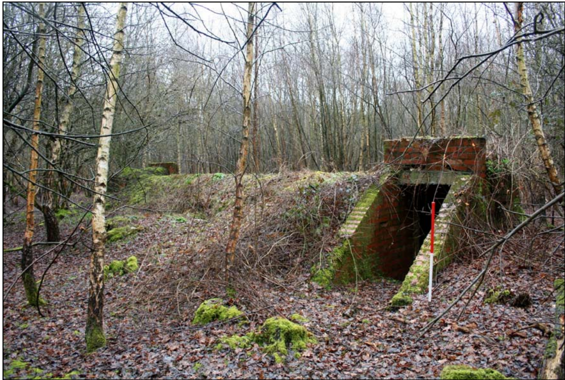
Plate 18: Example of a Stanton-type air raid shelter, Site 49
