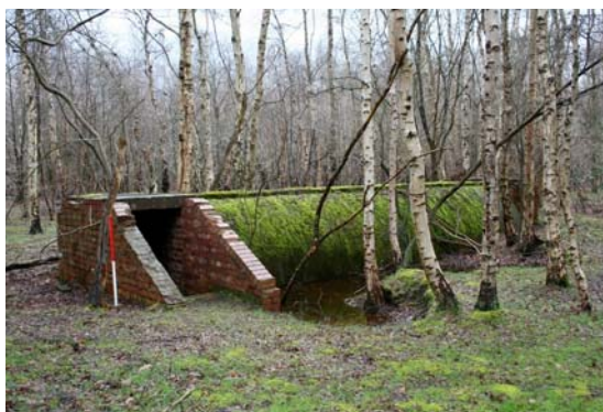
Plate 62: Air Raid Shelter, Site 279
