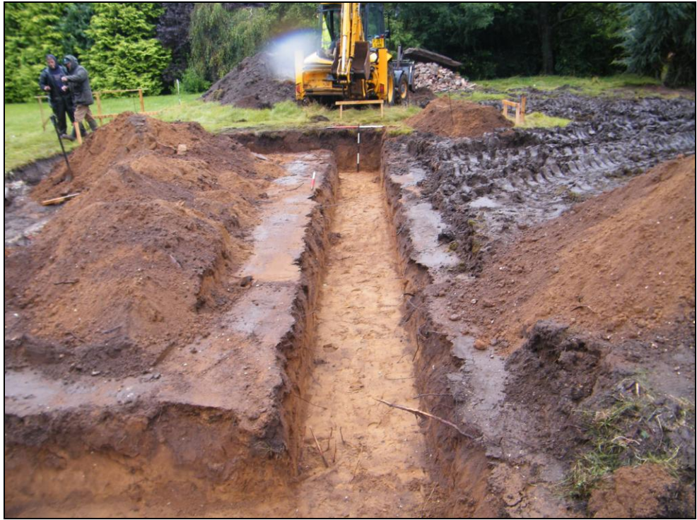
Figure 6: west foundation trench looking south
