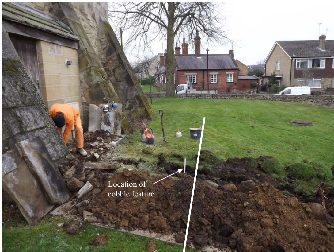
Plate 3. General view west showing break of slope associated with cobble feature
