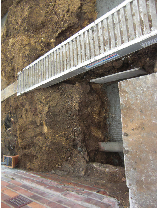
Plate 4. Services in Foundation Trench. Facing West.
