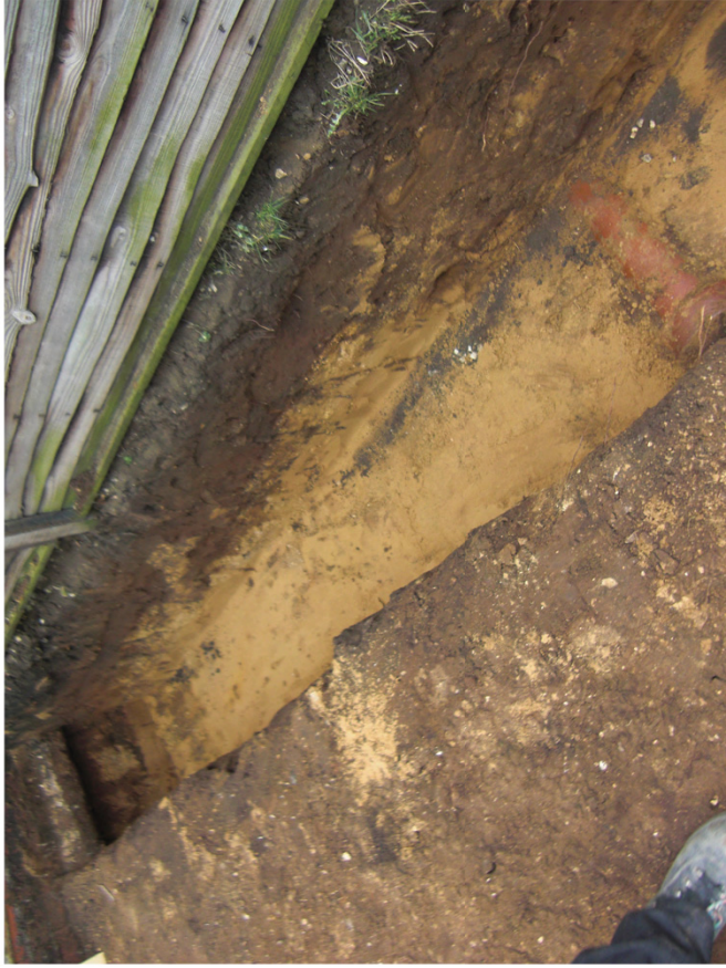
Plate 1. Founsdation Trench with Drain. Facing South-west.
