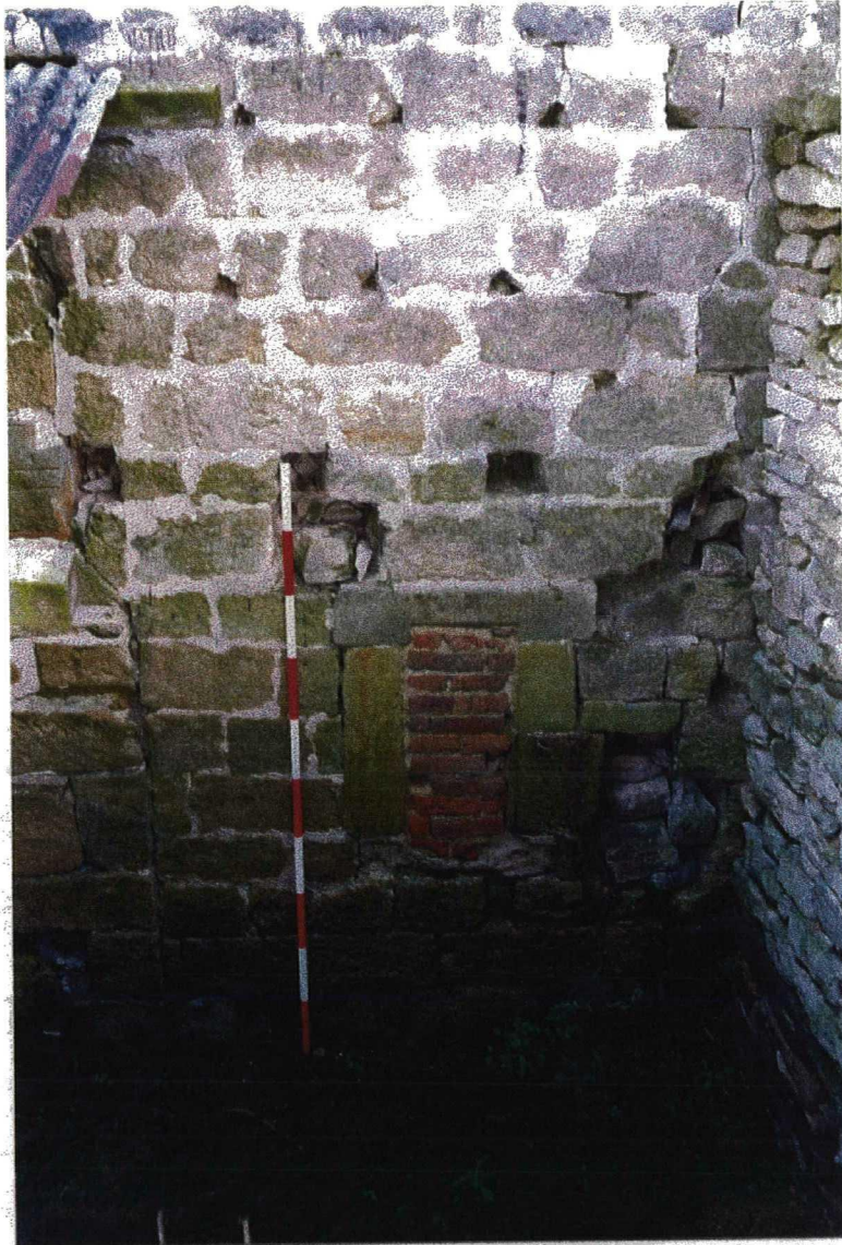
Plate 9. Fire Window. Facing South.
