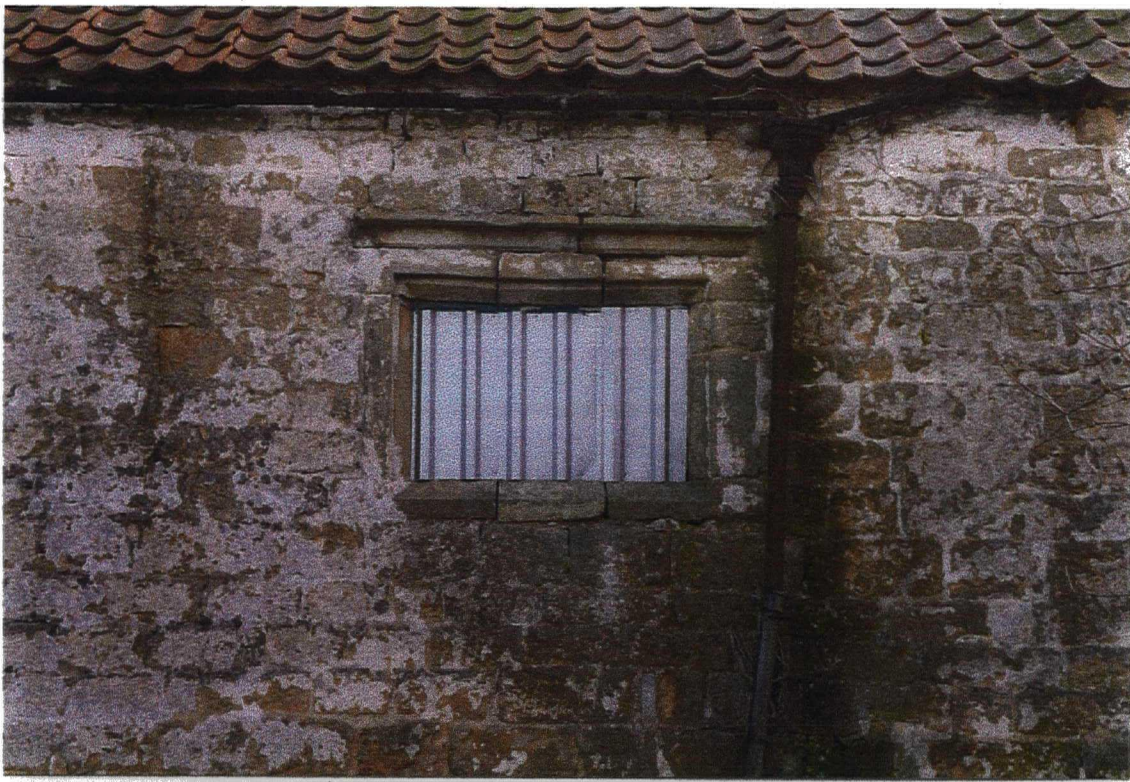
Plate 5. Late Seventeenth Century Window. Facing East.
