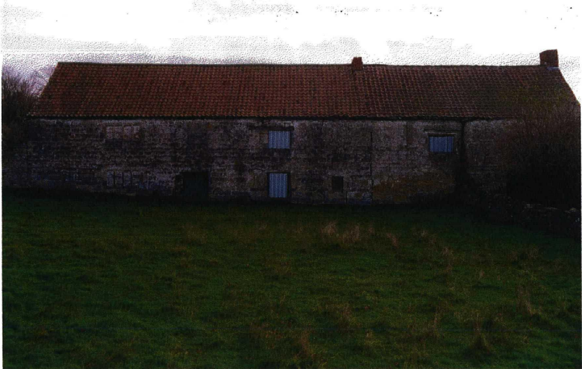
Plate 2. West Facade. Facing East.
