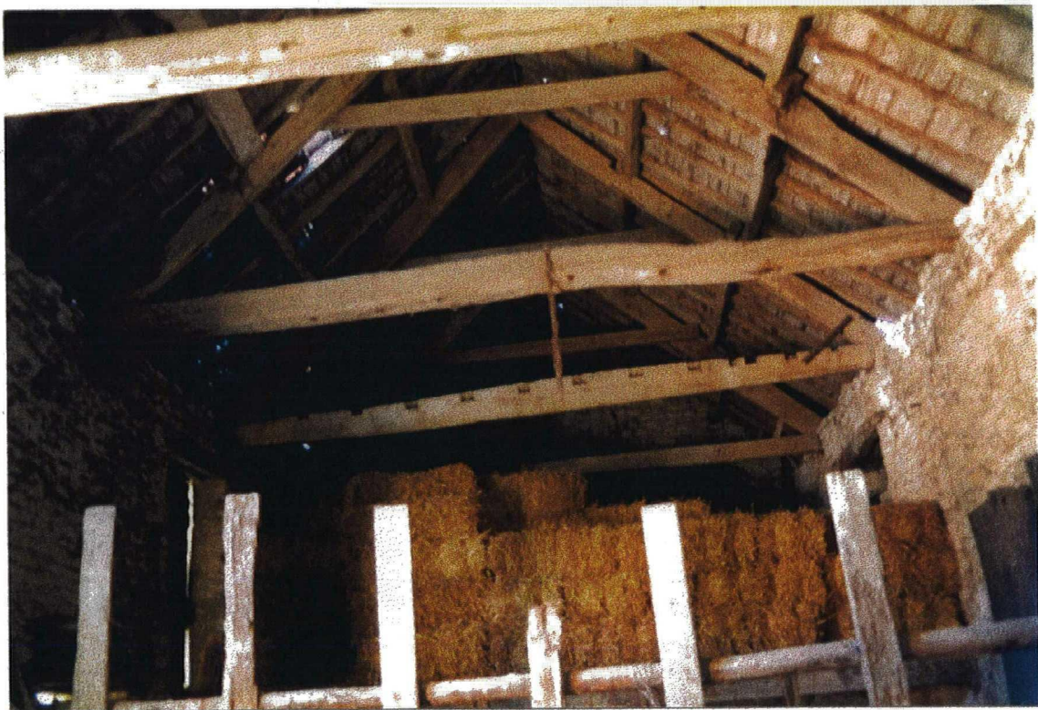
Plate 4. Barn Roof. Facing South.
