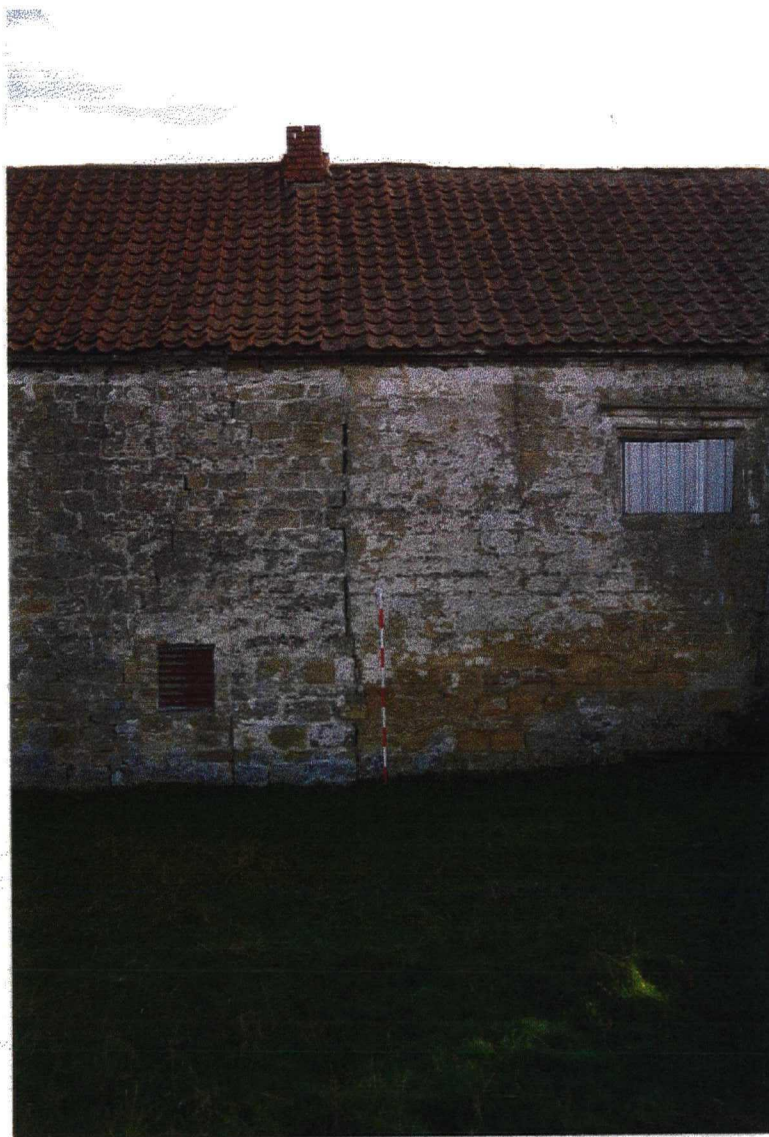
Plate 7. Blocked Door and Second Phase of Building. Facing East.
