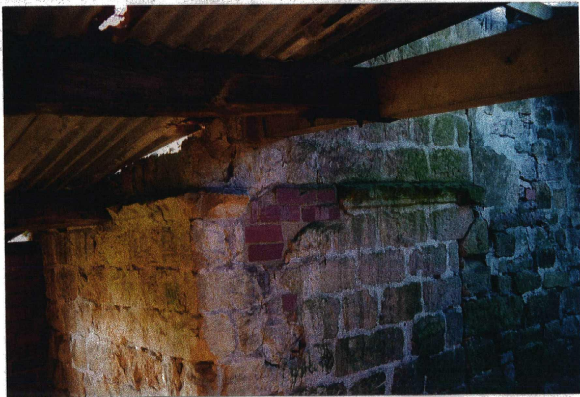
Plate 10. String Course in Northern Gable. Facing South-west.
