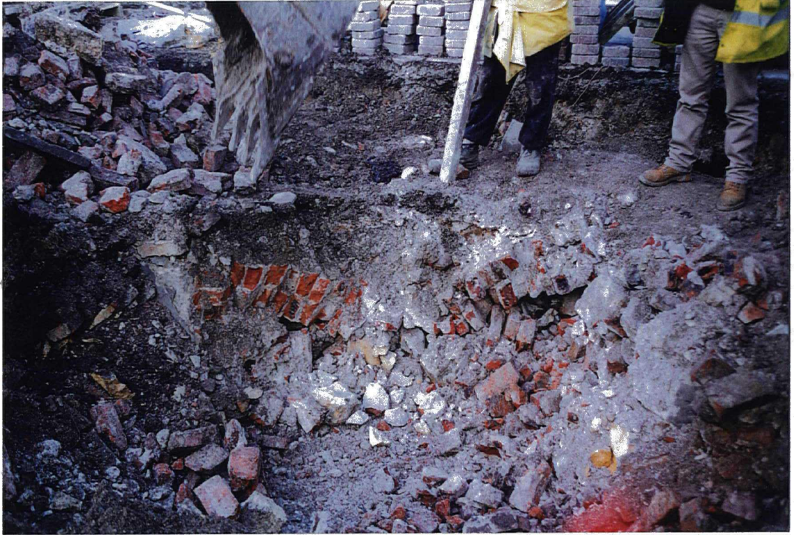
PLATE 1 Brick vaulting and remains of cross wall (looking north)
