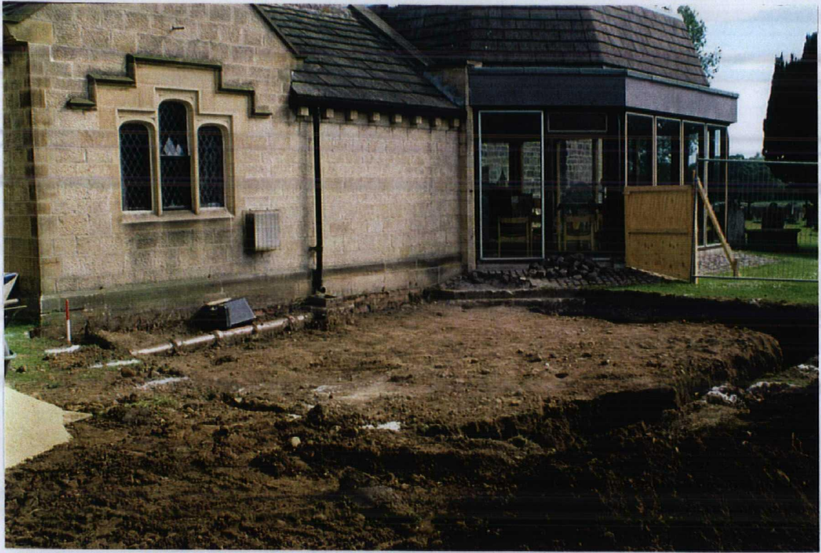
General site location on completion of foundation trench excavations.
