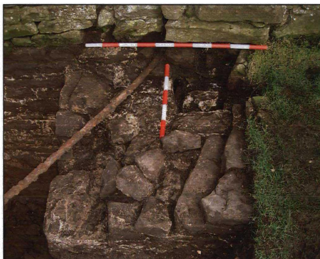
Plate 18: Trench 6: Chimney Stack [6015] and standing west wall of south range behind. Looking northeast.
