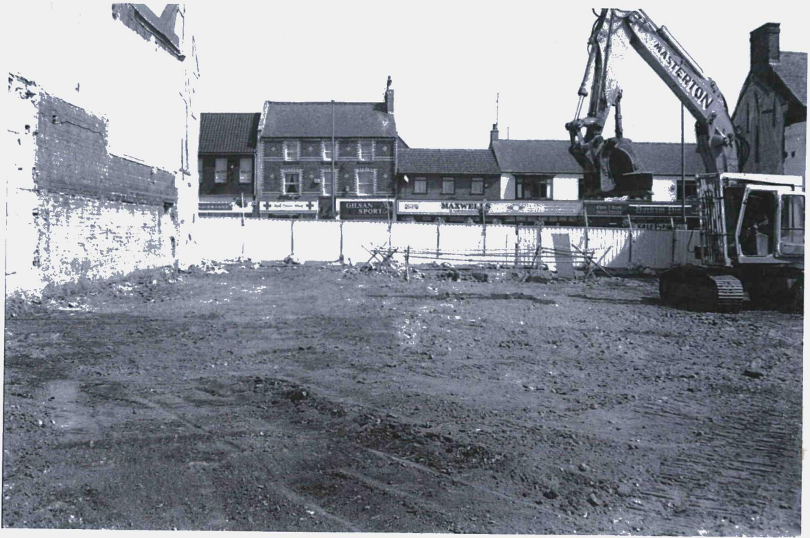
Plate 5 View to east after first levelling
