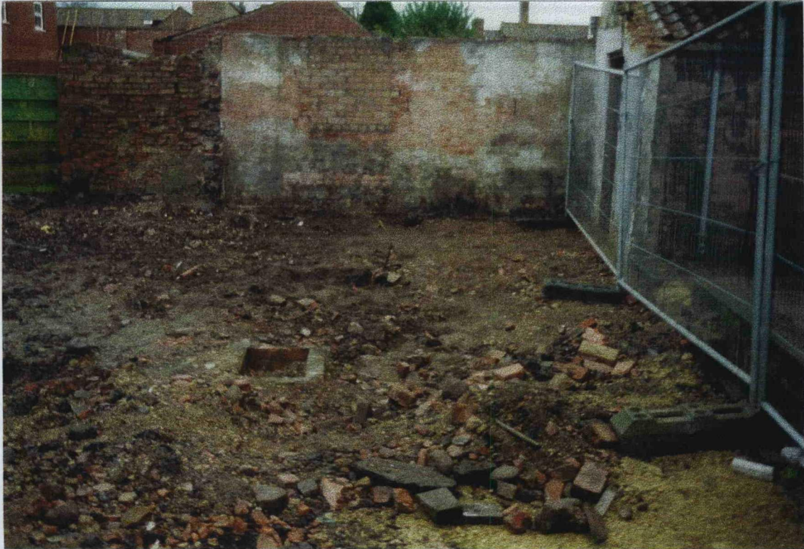
Plate 7. Area 2. After garage demolition. Facing east.
