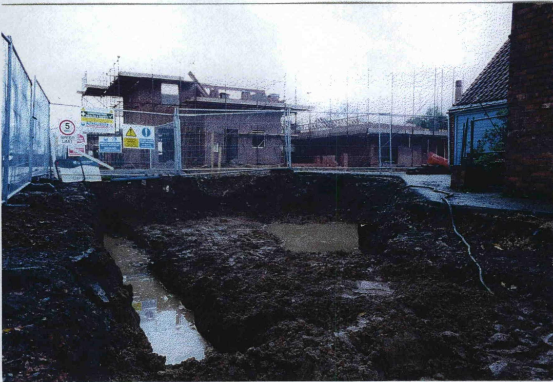
Plate 2. Area 1. After demolition. Facing north.
