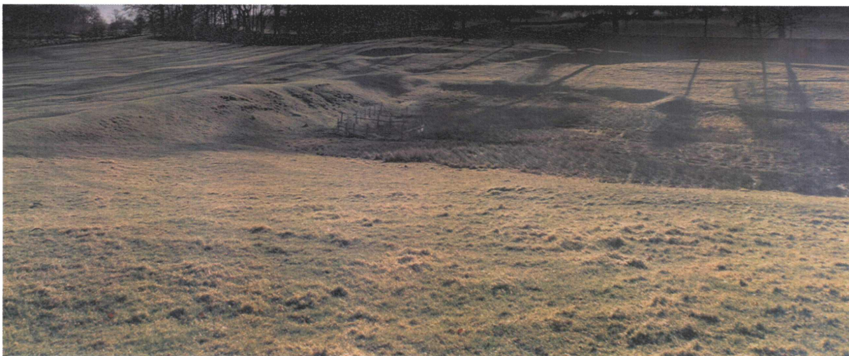
Figure 3. View across the monastic reservoir WF1, showing the dam DM1 (centre left) and to its right garden feature GS16 with building platform BC1 visible in the distance (NMR AA99/03571).
