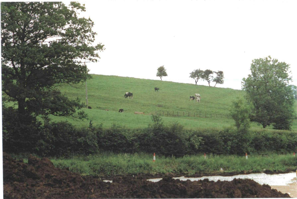
Plate 2. Earthworks to north-east of junction
