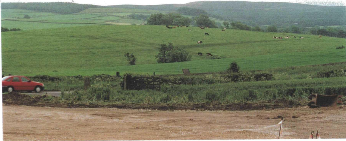
Plate 1. Earthworks to south-east of junction
