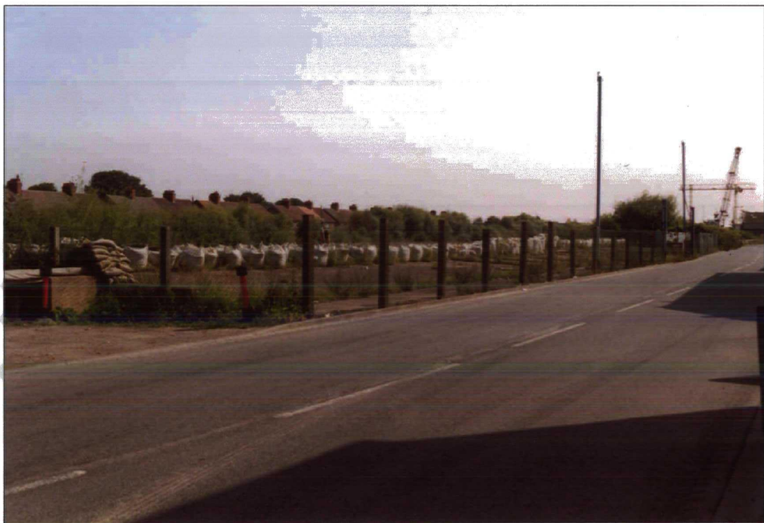
Plate 2 Wharf 2 (Area 5) looking east
