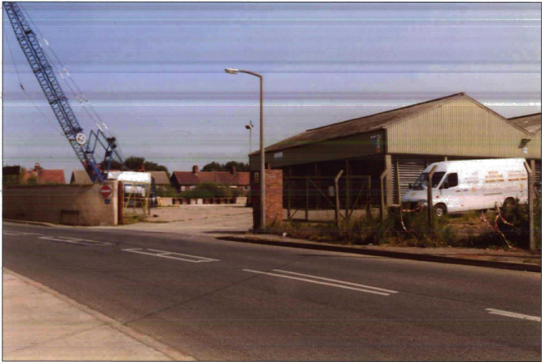
Plate 3 Area 2 looking north east
