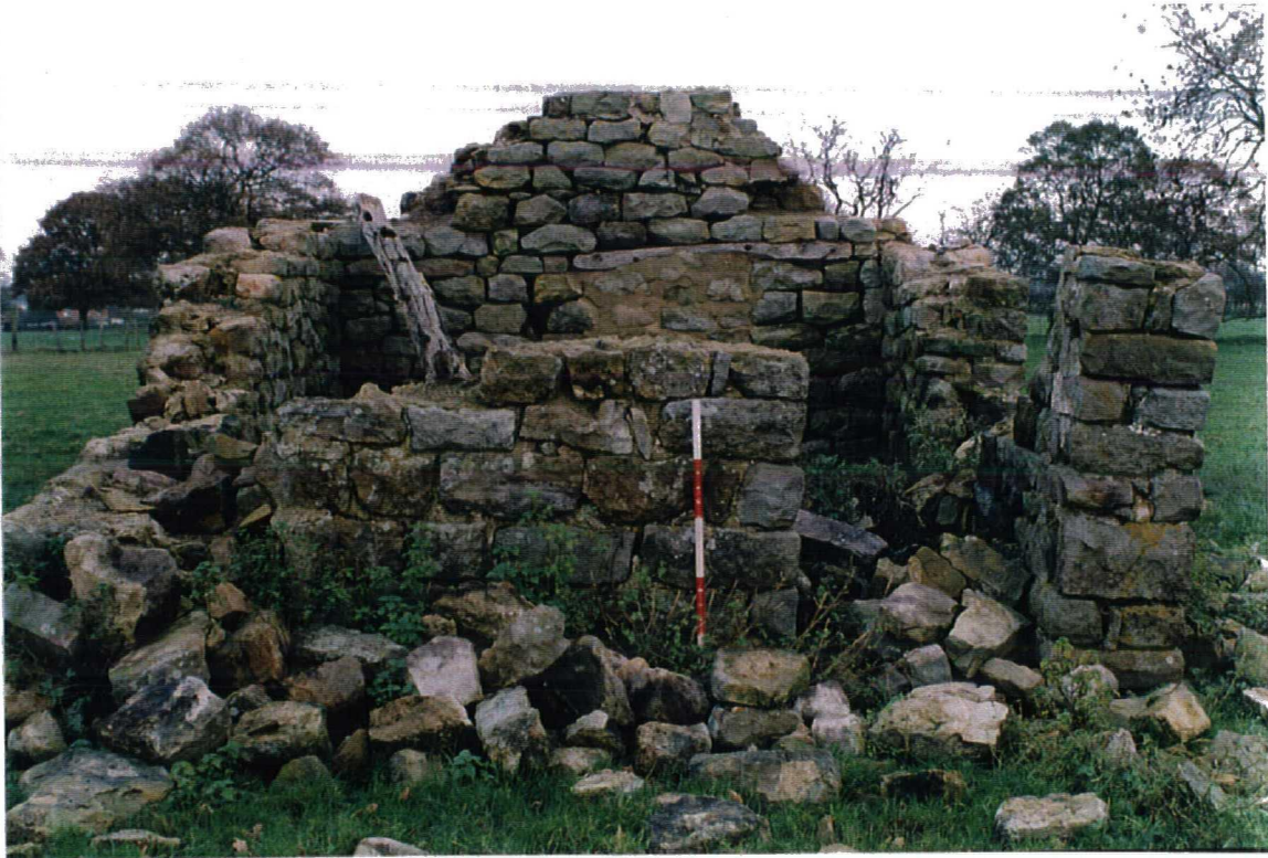
Field Barn, Record No.4840.0800, facing north east.
