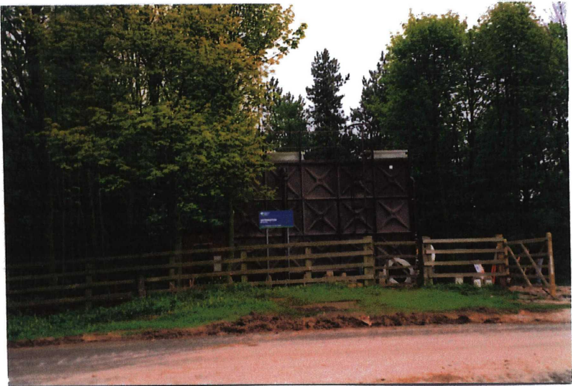
Plate 1. View of Site. Facing north.
