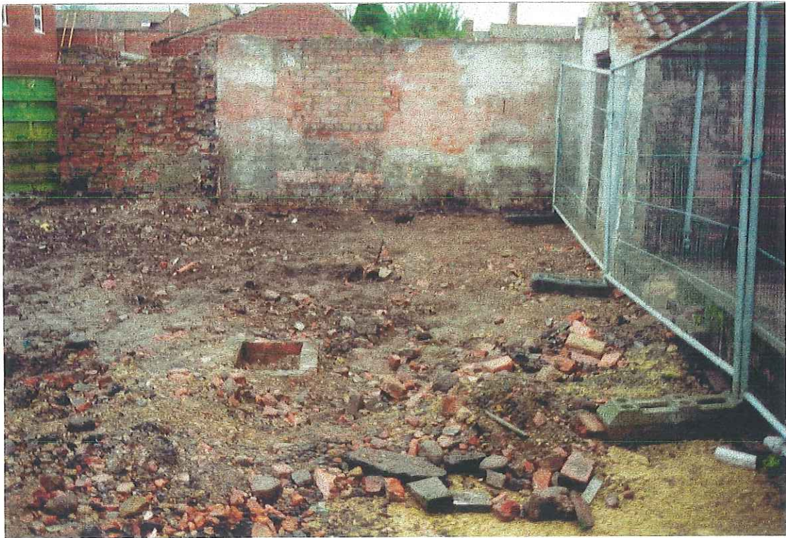
Plate 7. Area 2. After garage demolition. Facing east.
