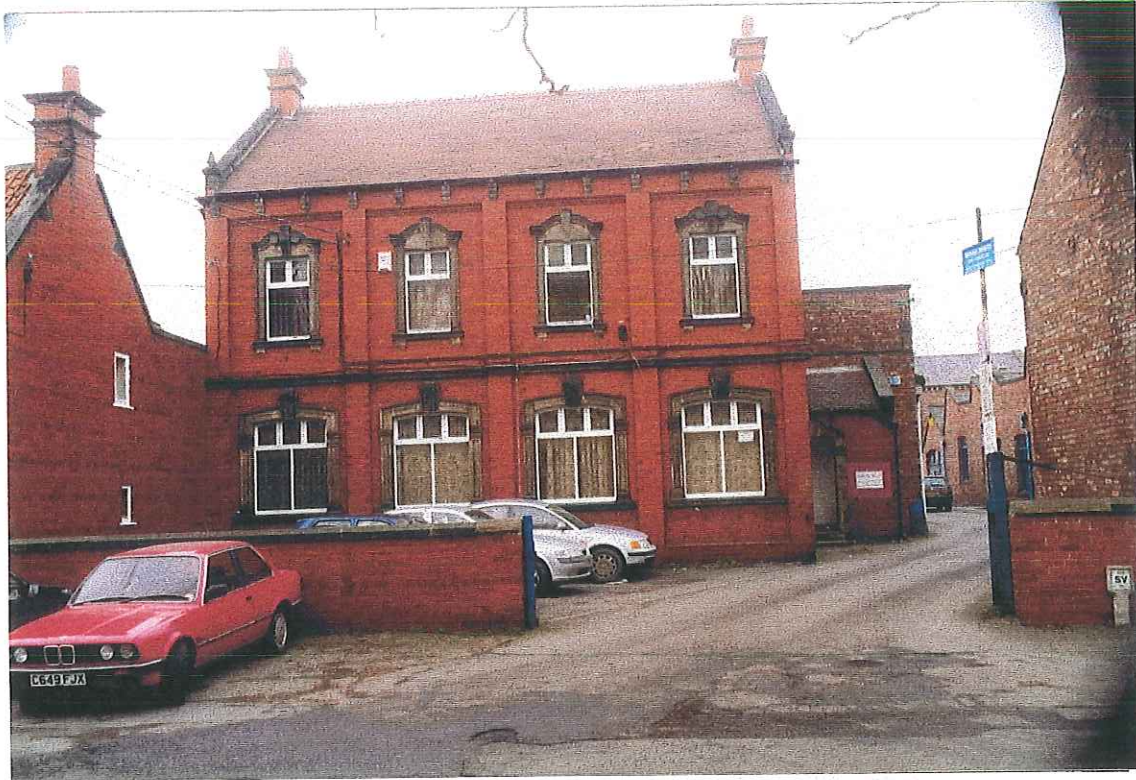
Plate 1. Area 1. View of Number 29 Church View. Facing north.
