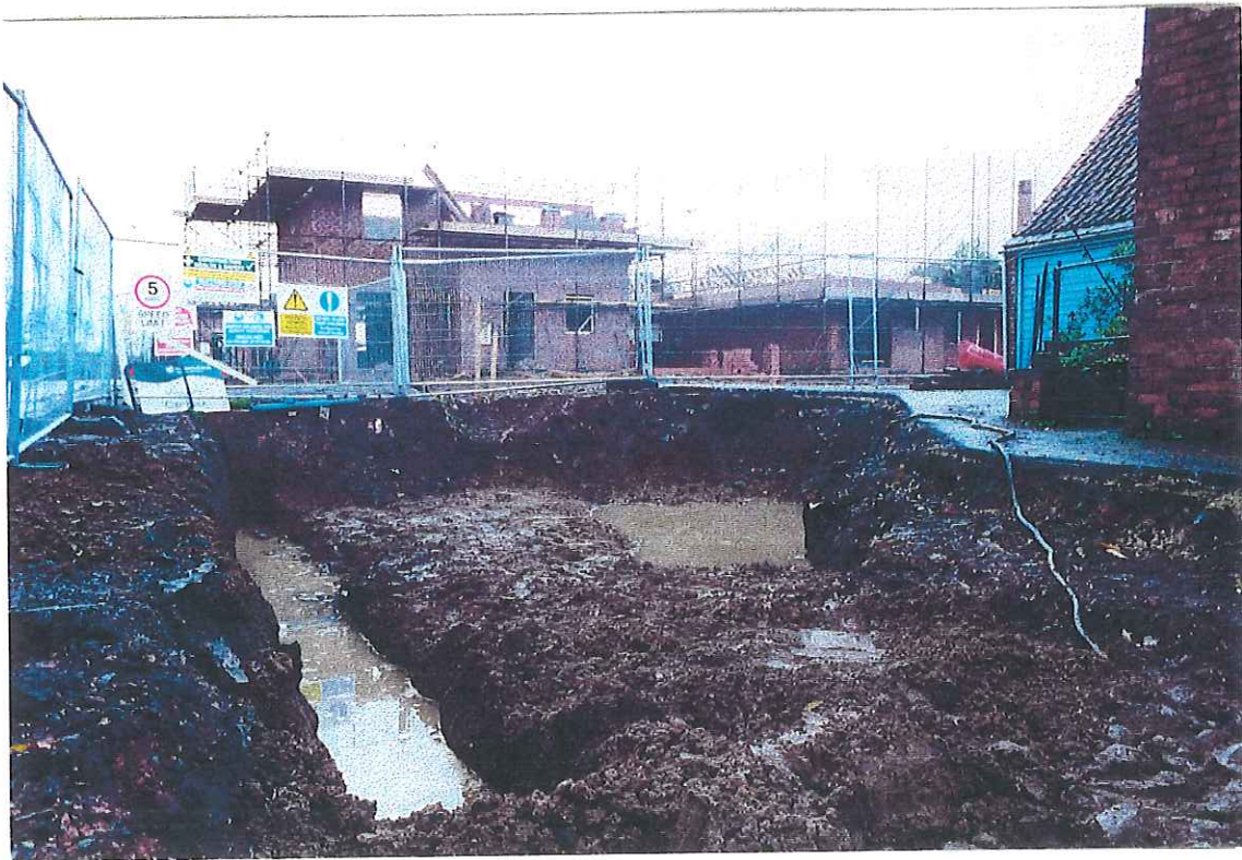
Plate 2. Area 1. After demolition. Facing north.
