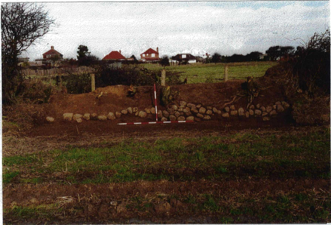
Plate 5. Cobble Revetting Wall 002. Facing North.
