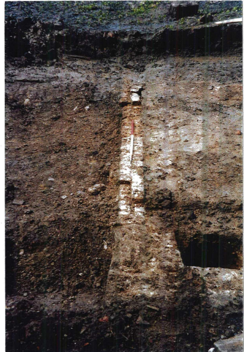
Plate 4. Wall 1005, constructed on Wall 1013. Facing Northwest.
