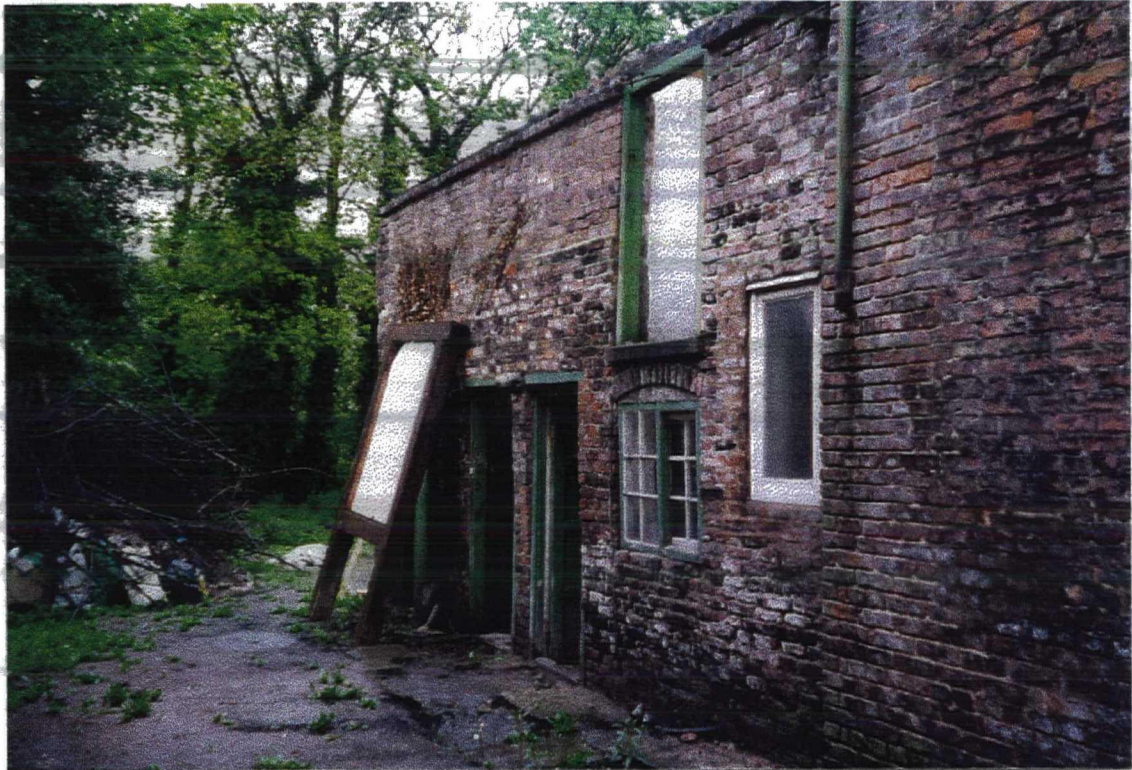
Plate 7. Rear of Brandsby House prior to Demolition. Facing South.
