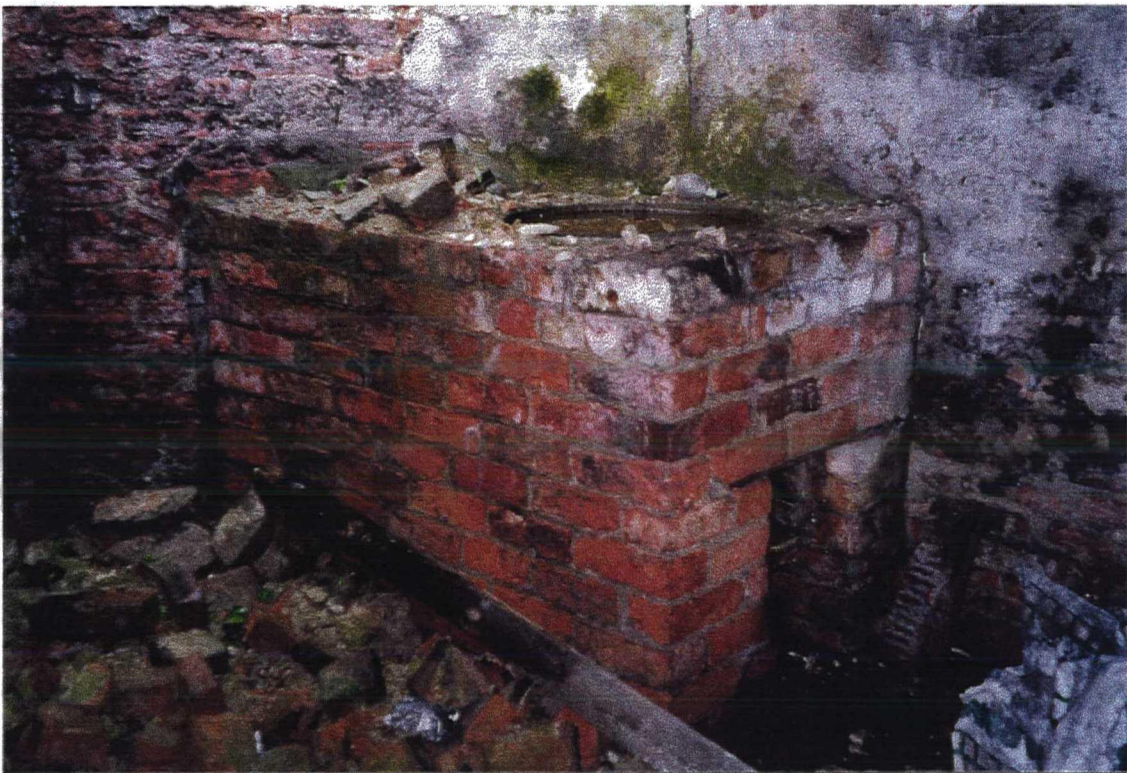
Plate 8. Nineteenth Century Copper in Scullery prior to Demolition. Facing South.
