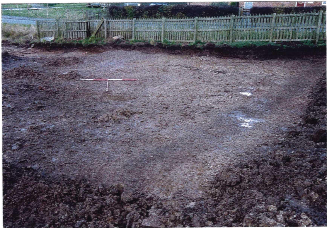
Plate 1. General shot of site prior to excavation. Facing north east.
