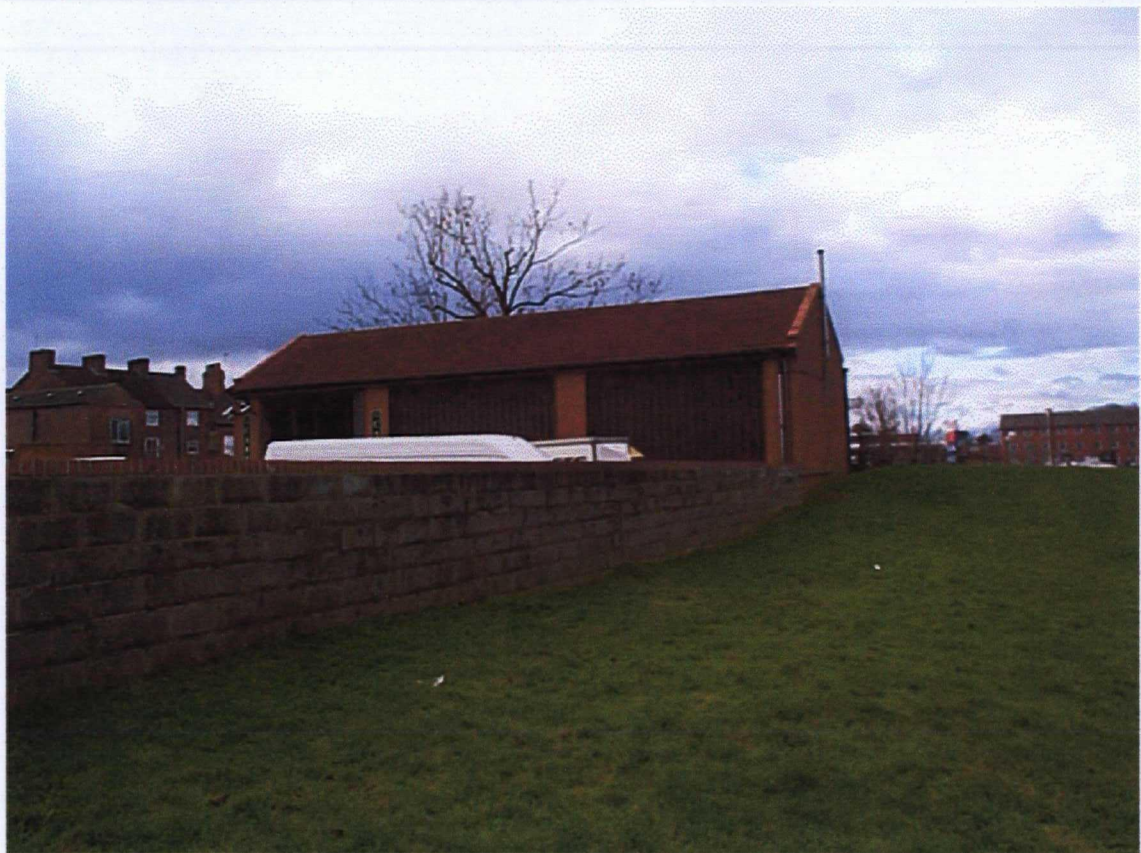
Plate 4. General view of site and Castle Garth. Facing south-west
