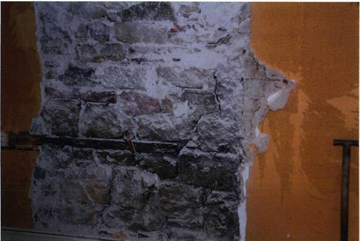
PLATE 6 NEW OPENING FROM EAST WITH DADO RAIL AND DATE STONE
