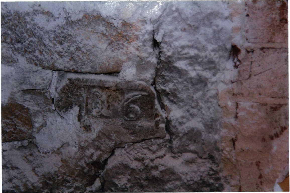
PLATE 9 DATE STONE SET INTO WALL
