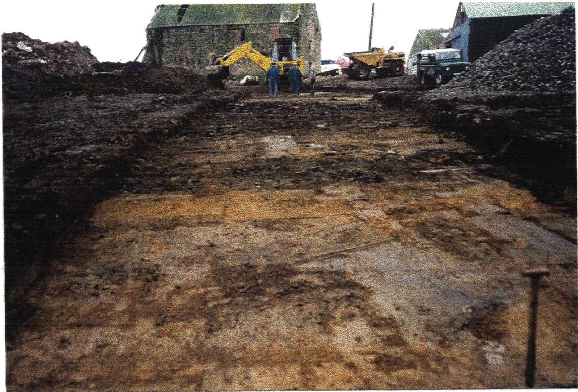
Plate 1. View of access road, after stripping. Facing north.
