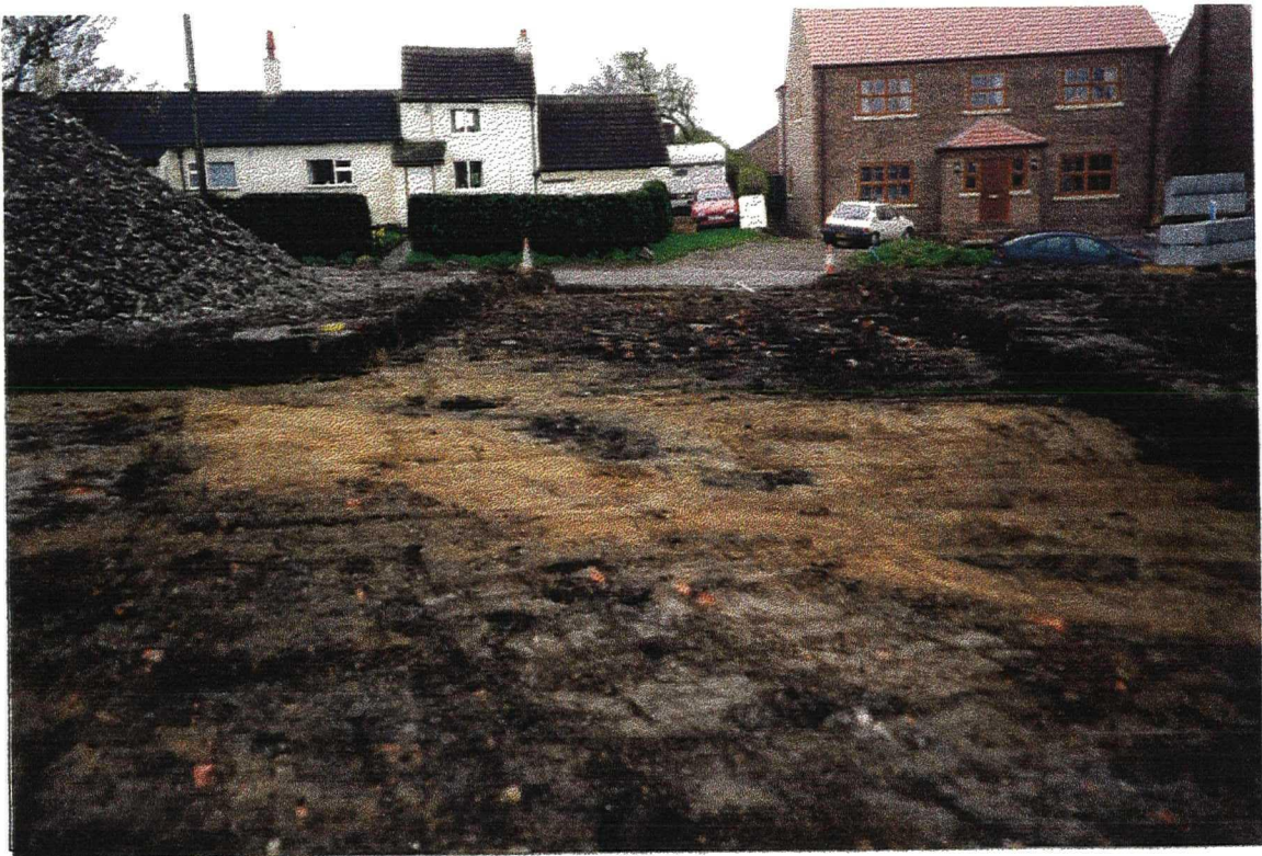
Plate 2. View of access road, after stripping. Facing south.
