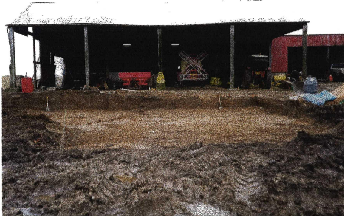
Plate 5. General view of Plot 8. Facing north.
