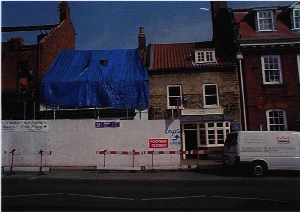
Plate 1. View of Nos. 40 & 42 Wheelgate. Street Frontage. Facing east.
