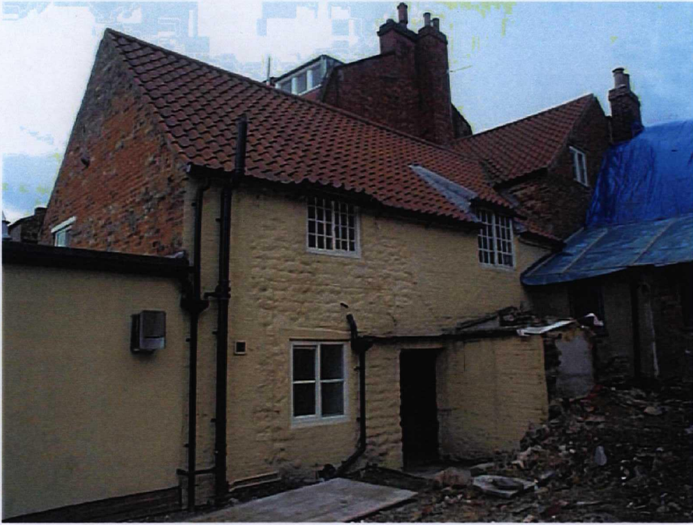
Plate 5. View of northern boundary to No. 46 Wheelgate. Facing north.
