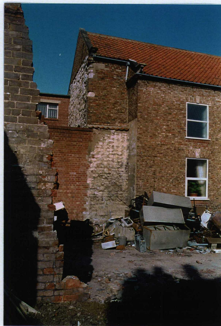
Plate 12. View of Stone Structure within Elim Church Building. Facing north.
