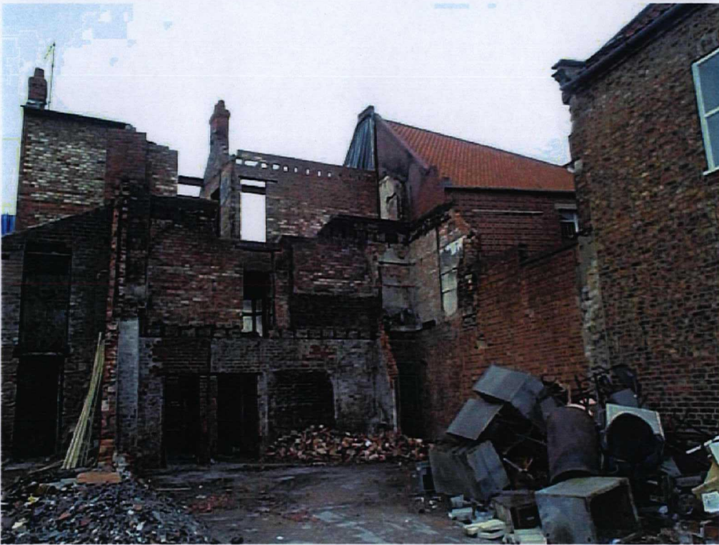
Plate 6. View of southern boundary to No. 42 Wheelgate. Facing south.
