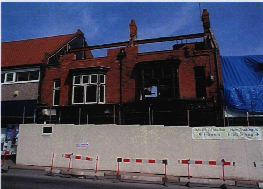
Plate 2. View of Nos. 44 & 46 Wheelgate. Street Frontage. Facing east.
