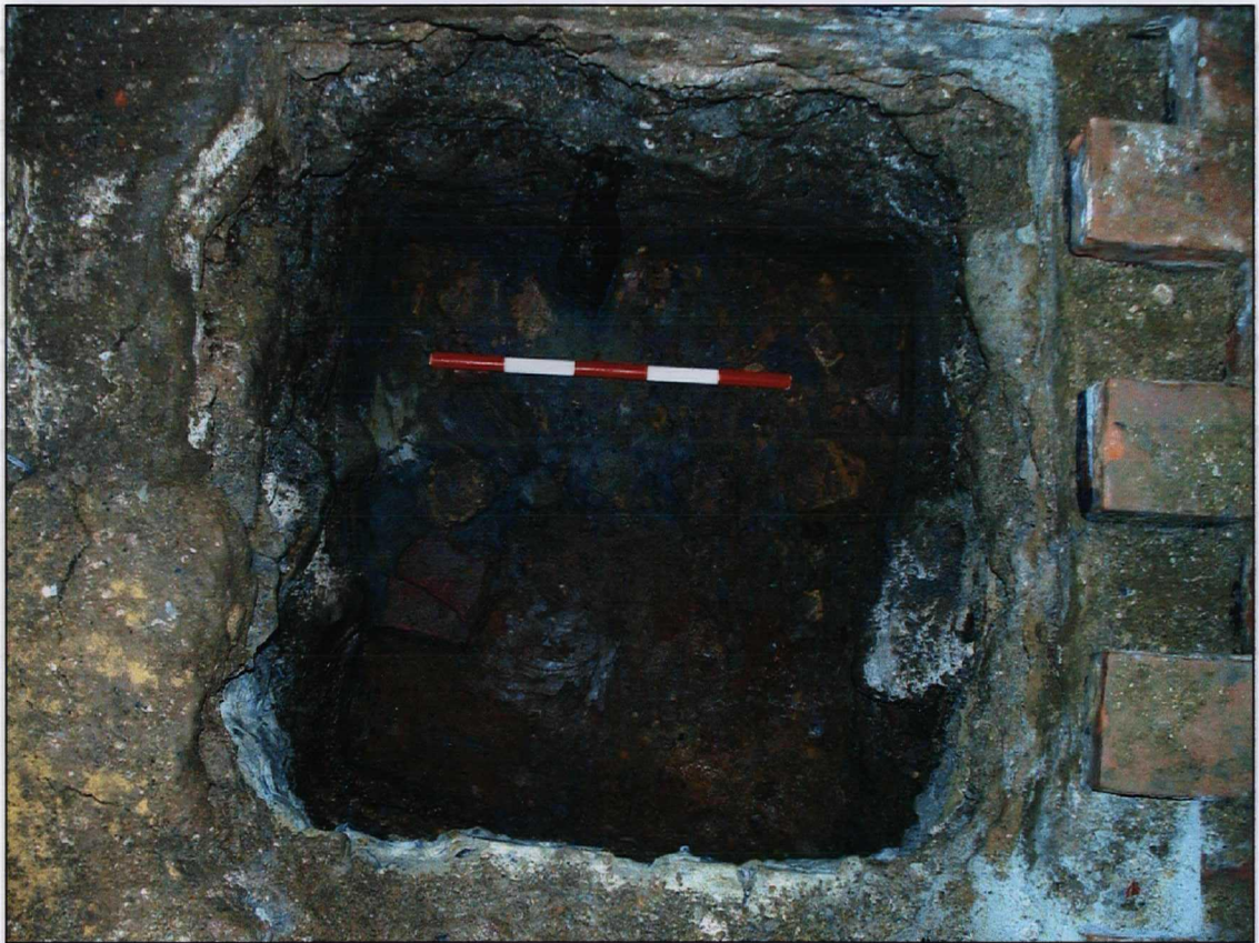
Plate 1. Foundation (116) and post (110). (Scale of 0.5m).
