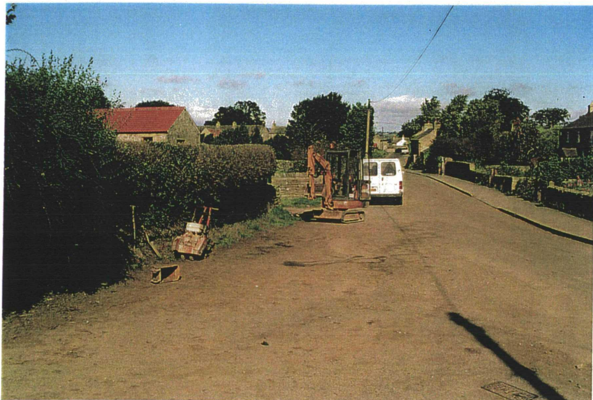
Low Thorpe Lane prior to groundworks, facing north.
