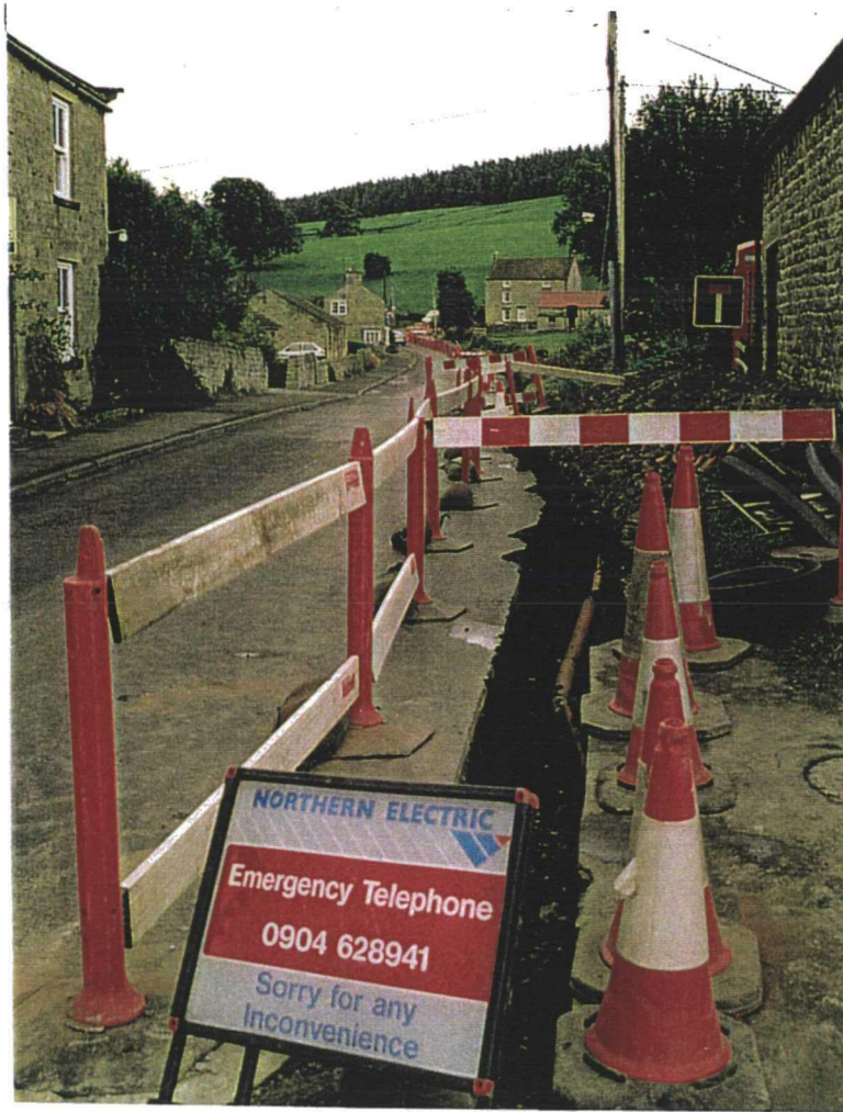
Low Thorpe Lane with Trench D excavated, facing south.
