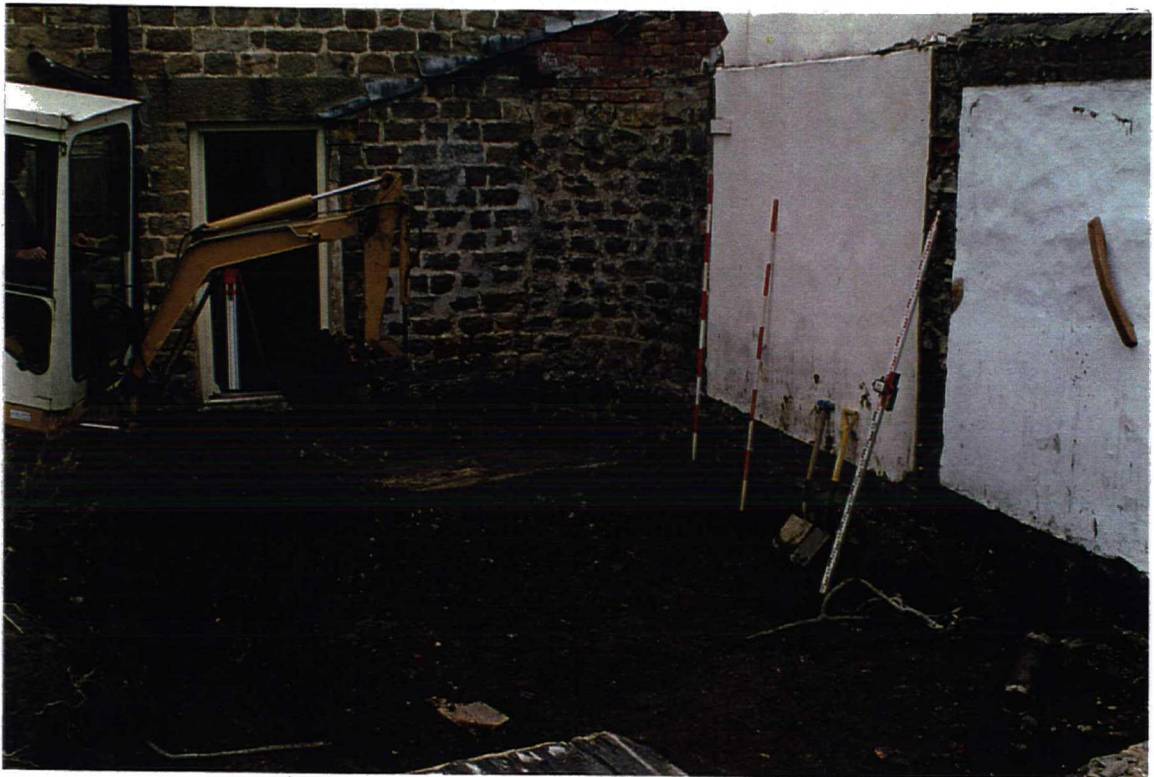
Site during excavation, facing north north east.
