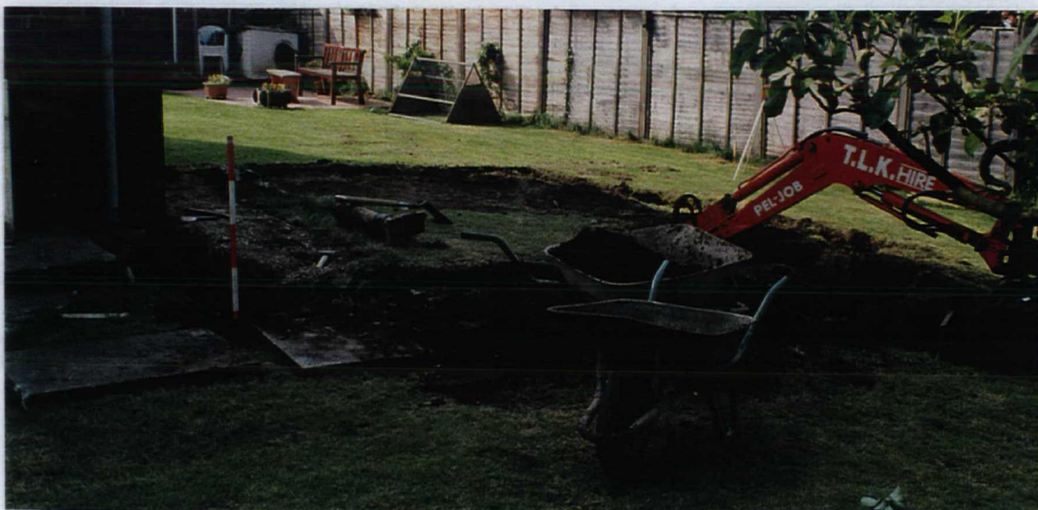
General site shot, following excavation, facing west north west.
