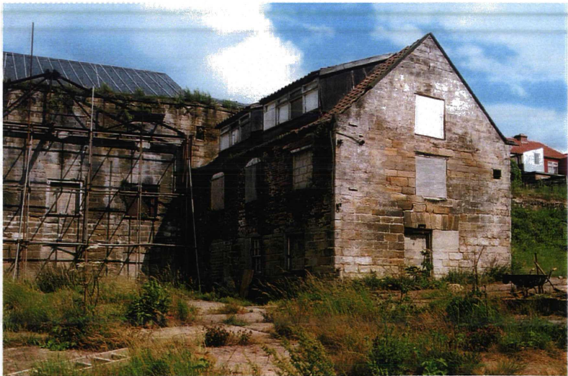
Plate 18. Old Sail Loft – long range and Sail Loft range from north-west
