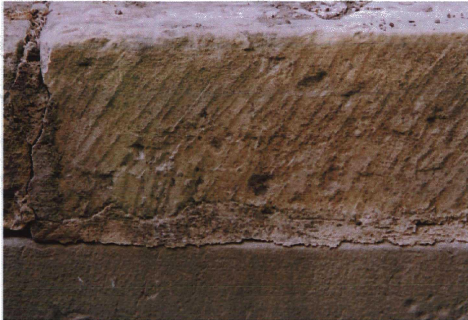
Plate 3 Tooling on kerb 1005
