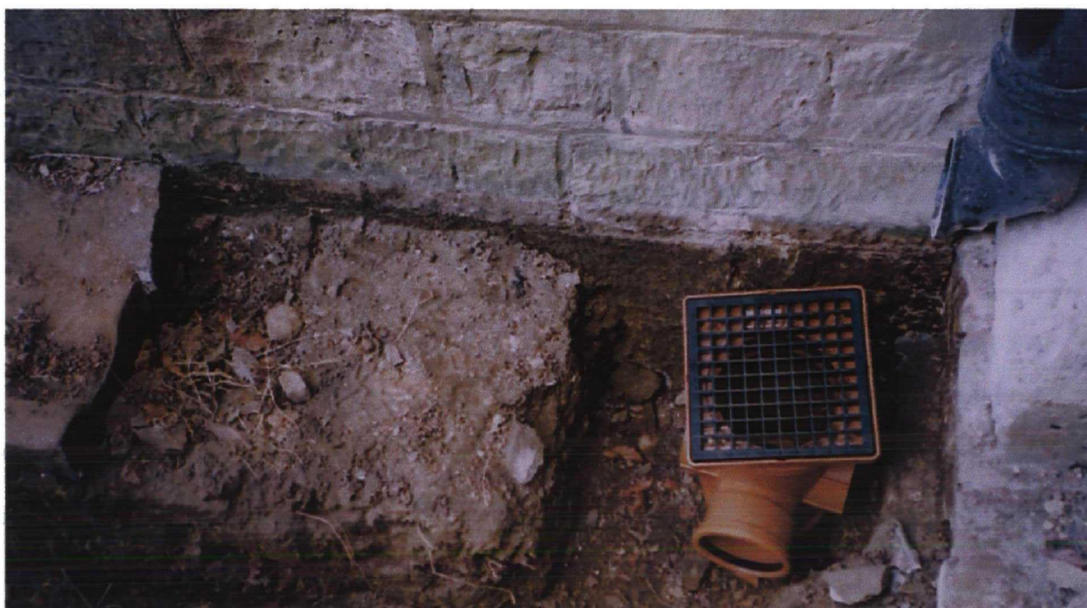
Plate 5 Church wall at junction of south aisle and chancel
