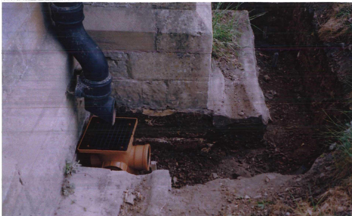
Plate 4 Footing of church wall
