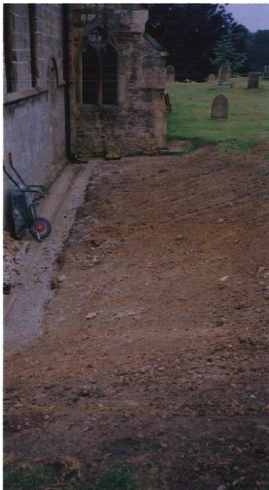
Plate 7 Grading down of cemetery soils to north of chancel
