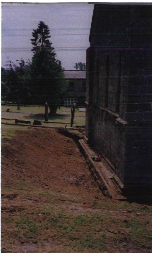
Plate 8 Grading down of cemetery soils to east of chancel
