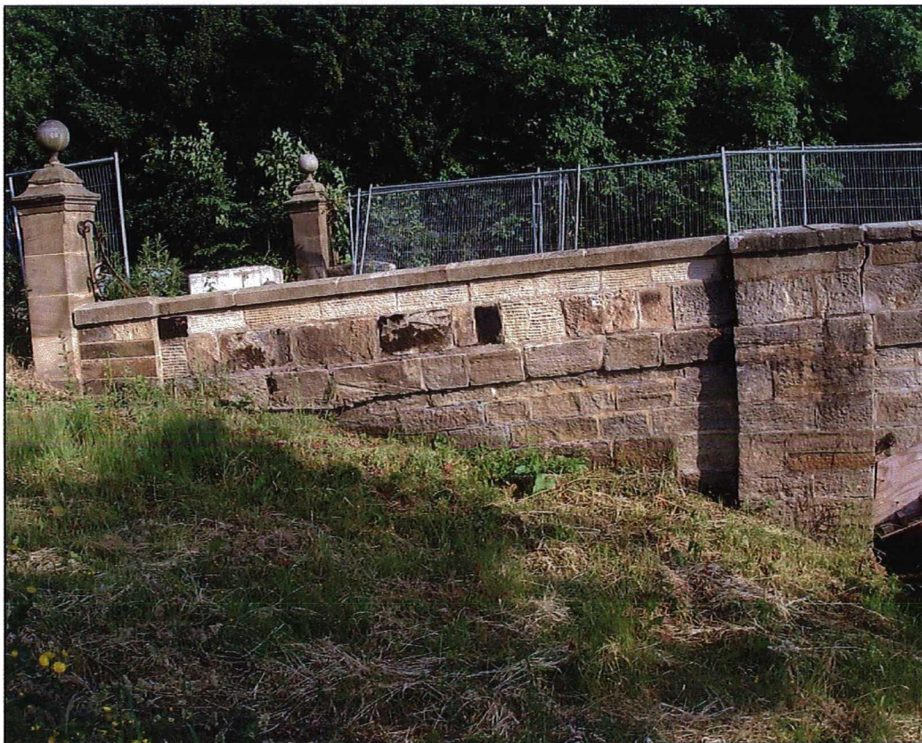
Plate 8. Southwest wing wall (1002) shown buried by made up ground (1004).
