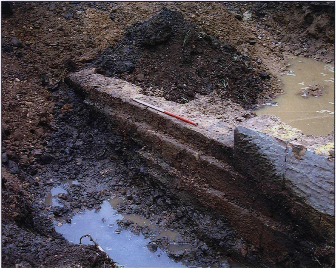
Plate 3. Southwest masonry base for abutments (1012), stepped into bank. (Scale of 1m).
