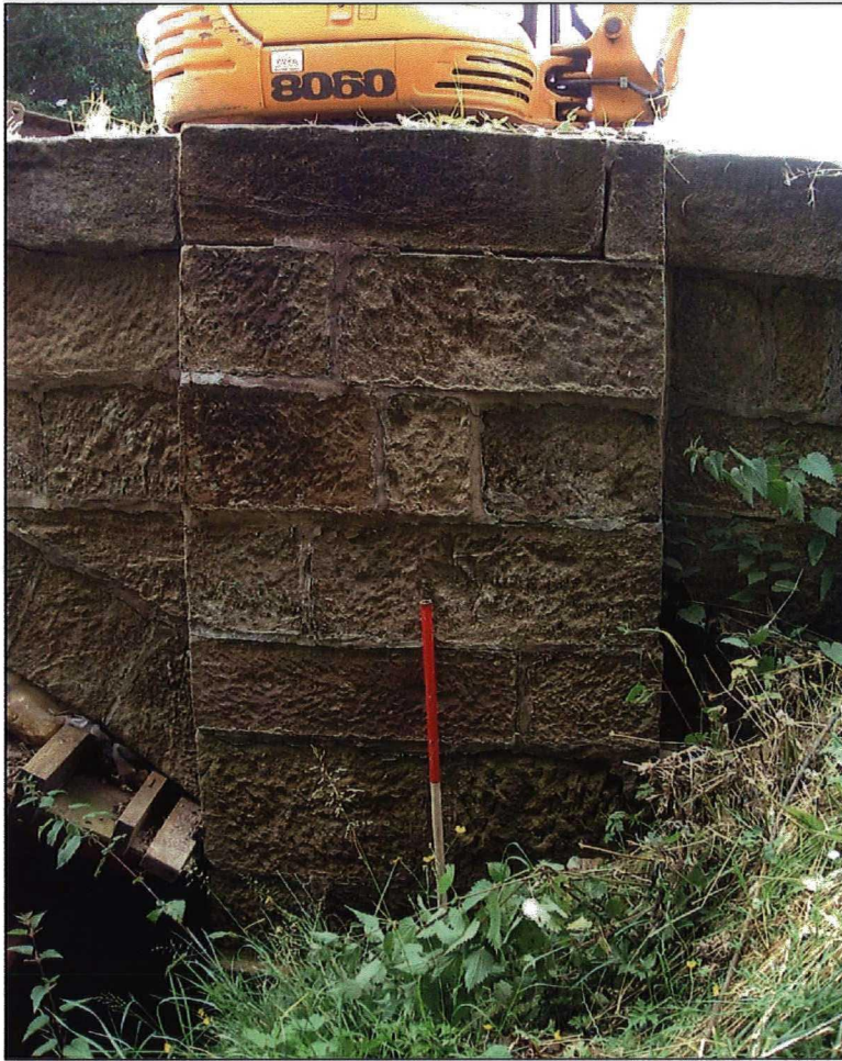
Plate 7. Northwest abutment masonry (1014). (Scale of 1m).
