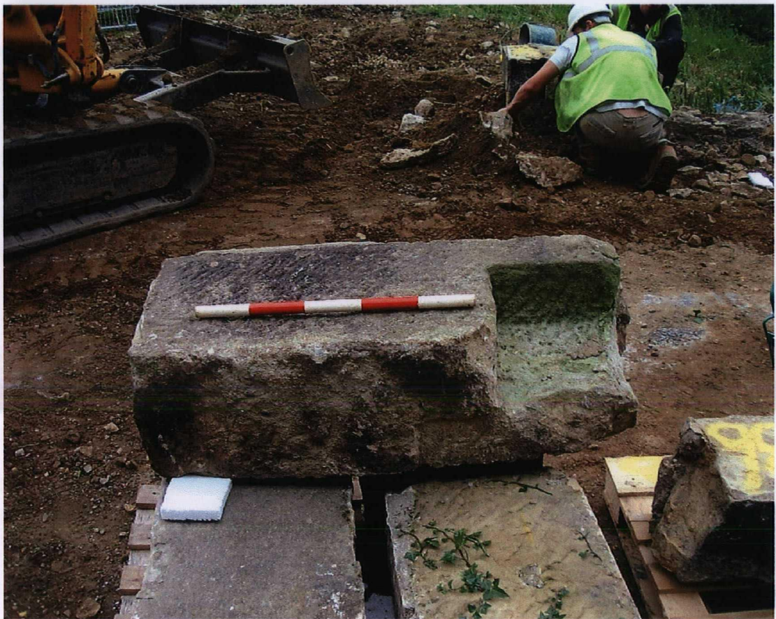
Plate 12. Removed masonry from parapet. (Scale of 0.5m).
