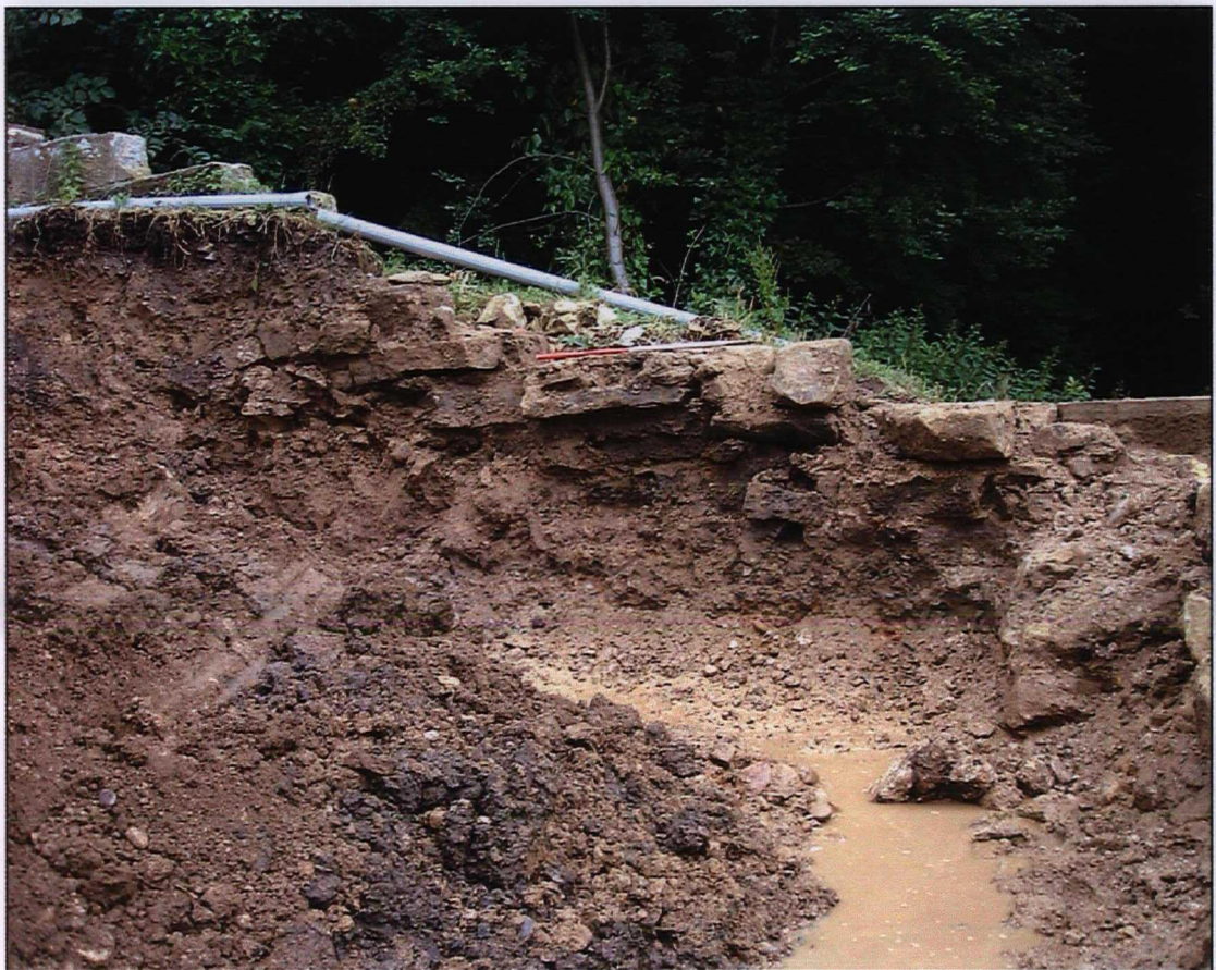
Plate 4. Northwest masonry base for abutments (1012), stepped into bank. (Scale of 1m)..
