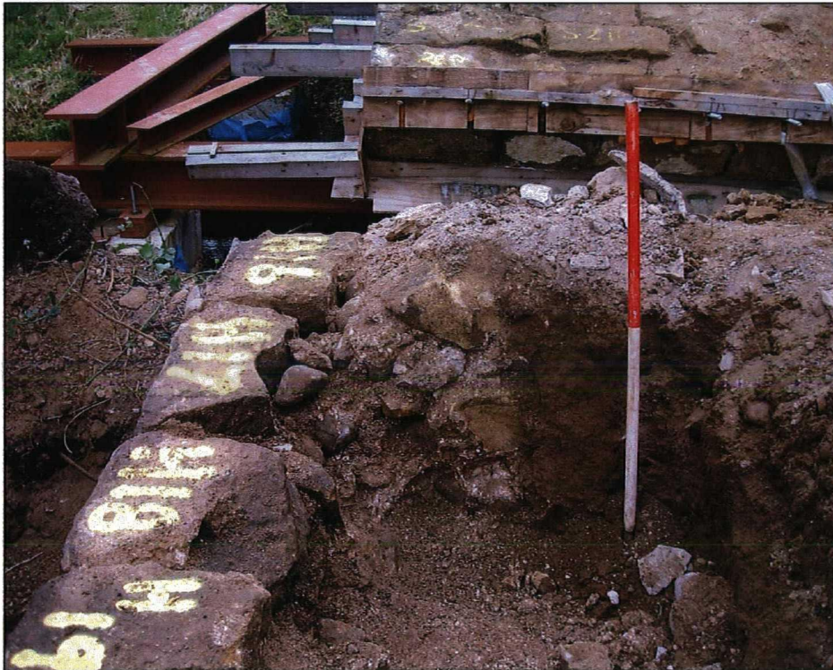
Plate 14. Lime mortar, cobble and sandstone fragments, backing to southeast wing wall, (1011). (Scale of 1m).
