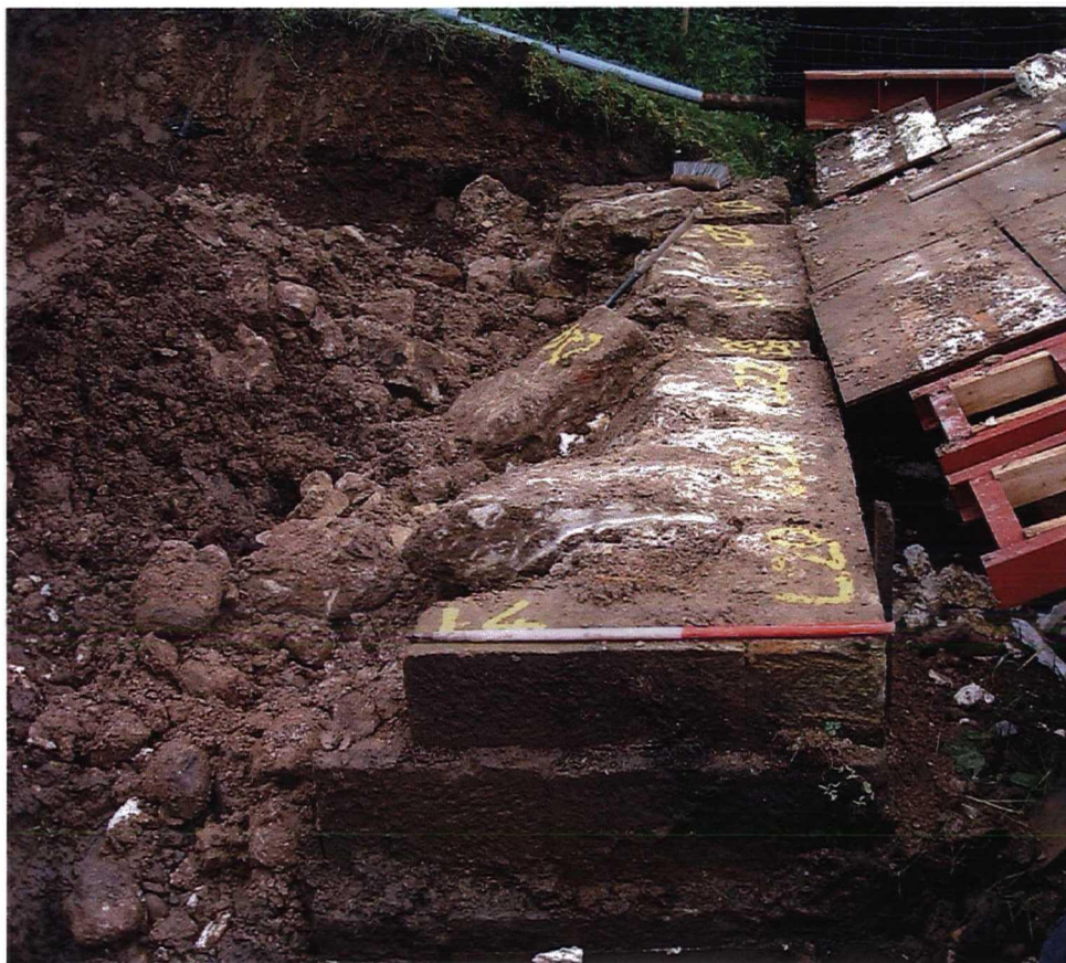
Plate 2. West masonry base for abutments and wing wall (1012). (Scale of 1m).
