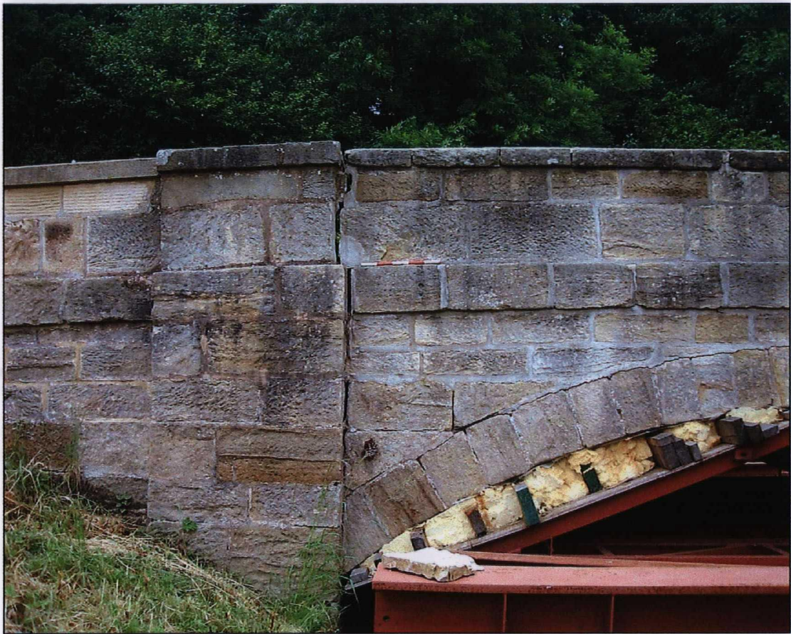
Plate 11. Spandrel masonry (1002) above bridge arch. (Scale of 0.5m).
