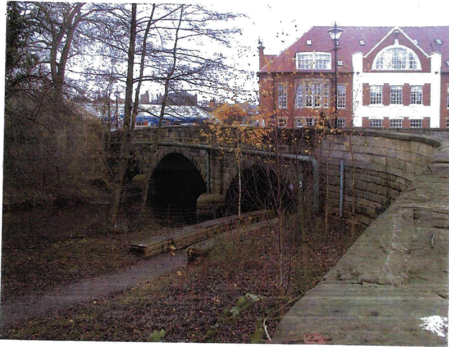
Plate 14. Borrage Bridge, west side
