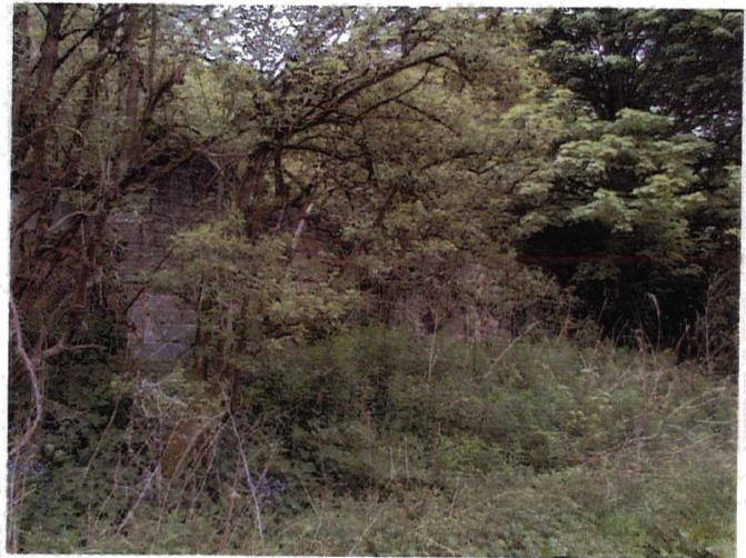
Plate 8, South side of building range close to Aldfield Spa
