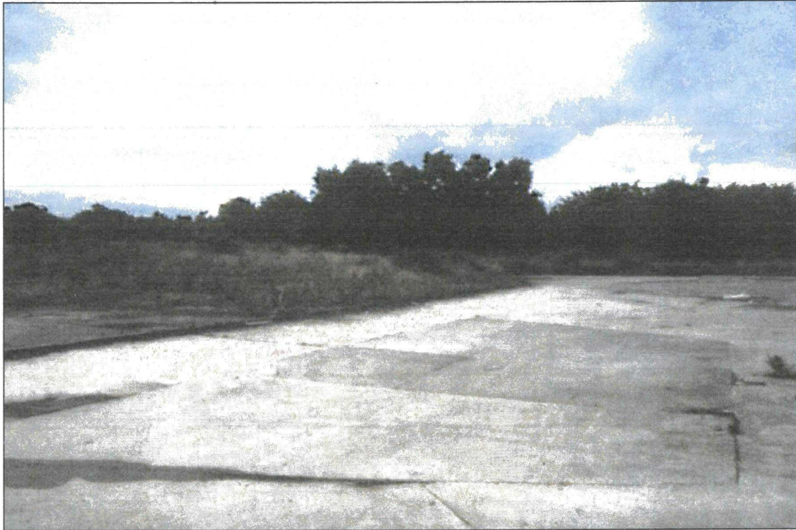
Plate 3 Earthwork to South-West of CAMAS factory (from the East)
