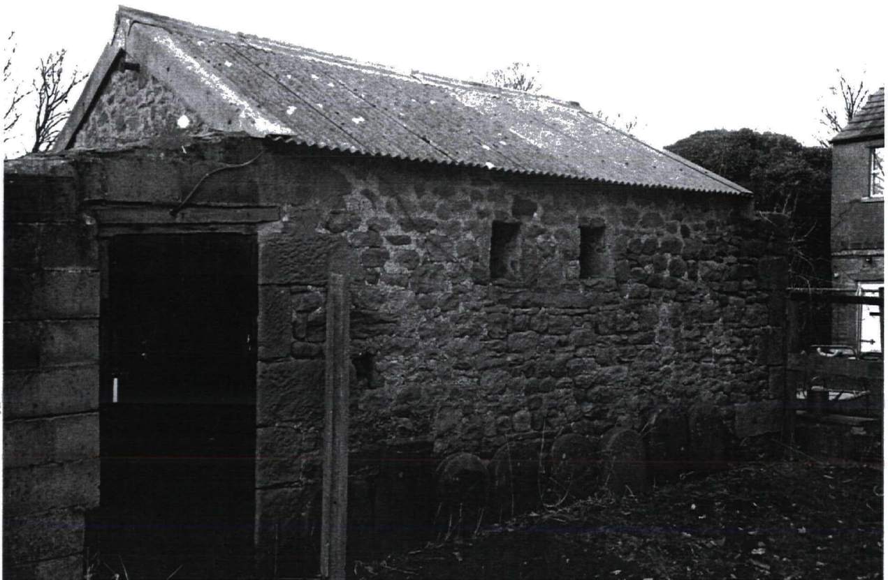
Plate 2. East elevation of Game Larder, showing quoins and ventilators
