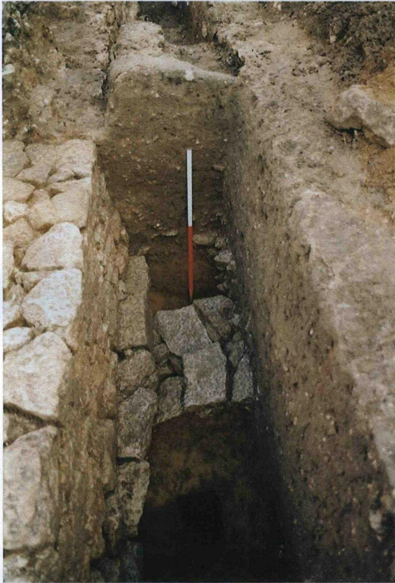
Plate 1. Limestone pit fill 038 and offset course of wall 028. Facing west.
