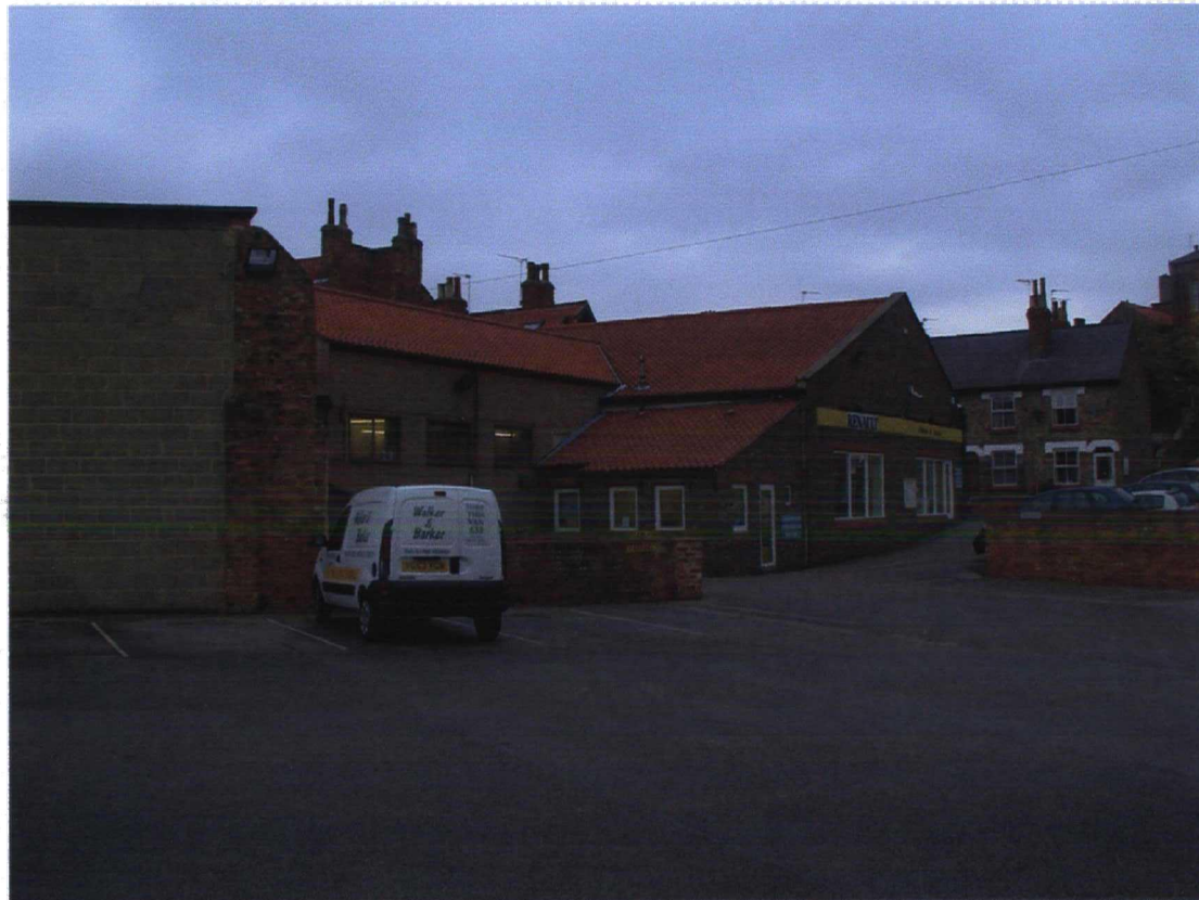
Plate 4 North-west part of site. Looking north-west
