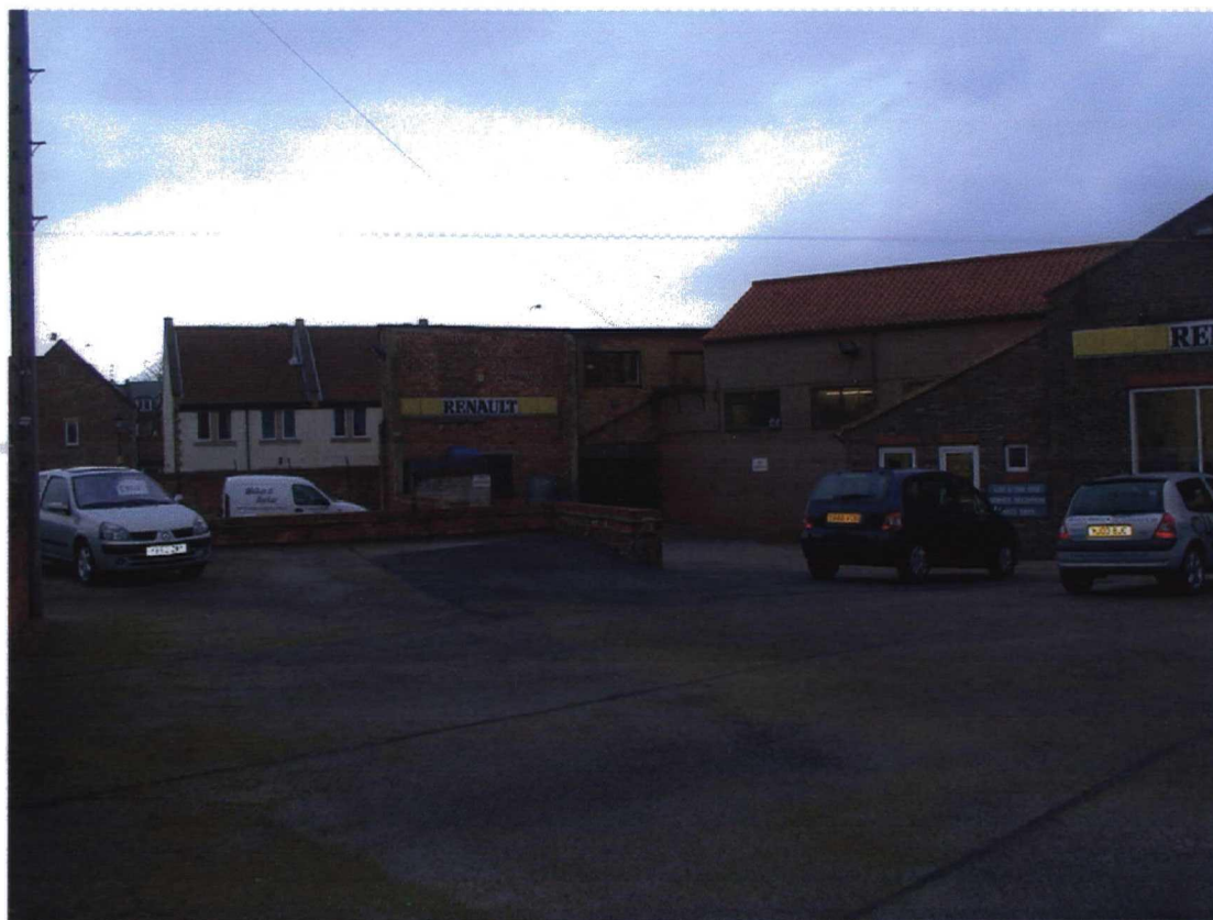
Plate 1 Workshops in south-west corner of site. Looking south-west
