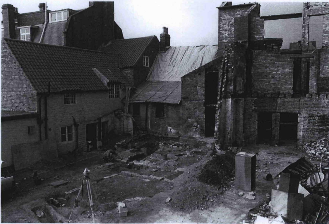
Plate 1: General View of Site. Facing South-west.
