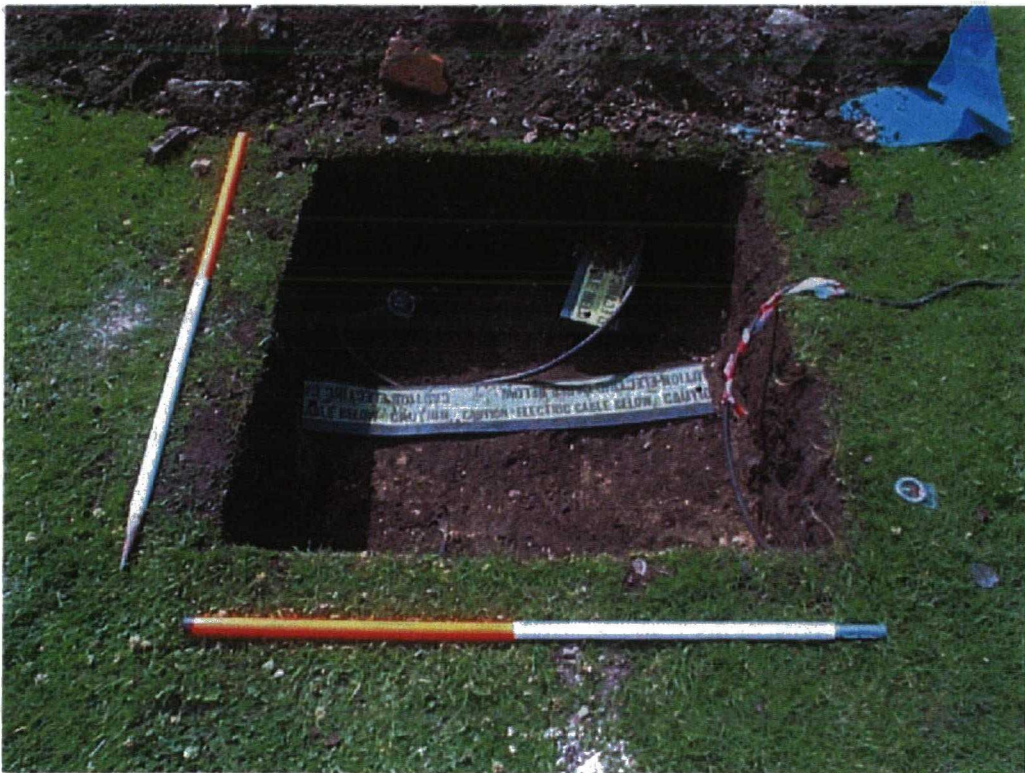
Plate 2. Trench 2. Facing South West
