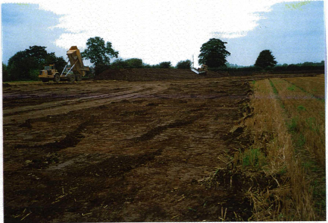
Plate 3. View of site during stripping. Facing north-west.
