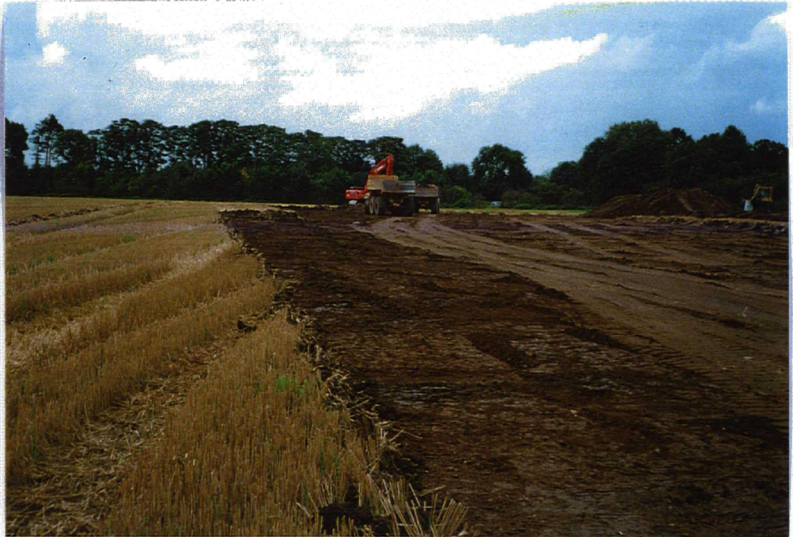
Plate 1. View of site during stripping. Facing north-east.
