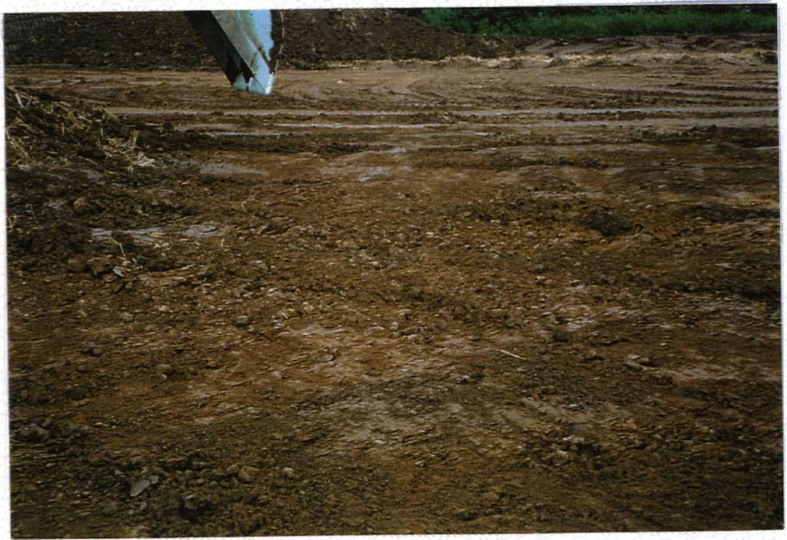
Plate 4. View of site during stripping. Facing east.
