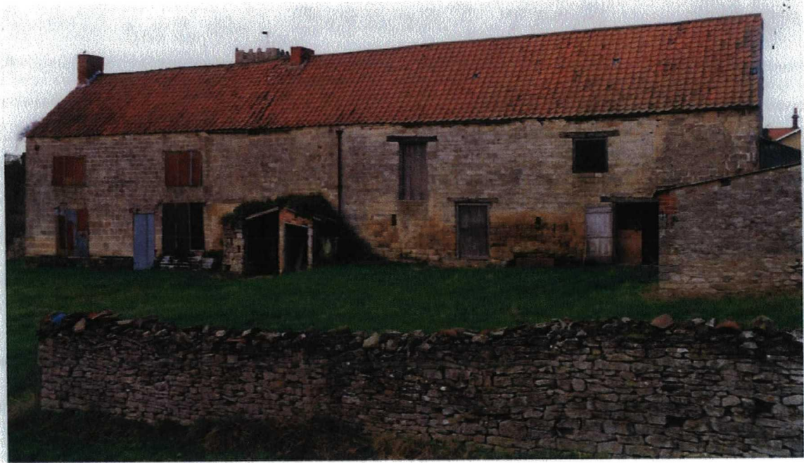
Plate 1. Exterior of Church Farm. Facing West
